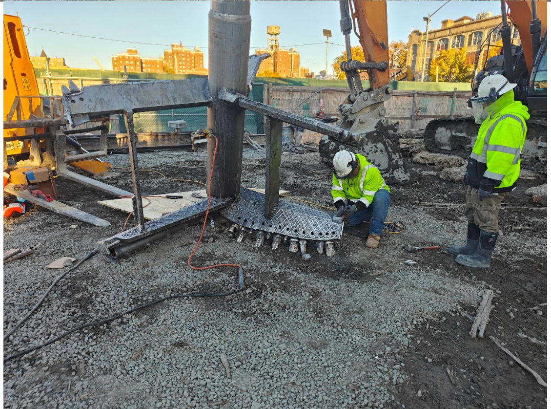
Photo 4- Representative Photo of augur maintenance.
