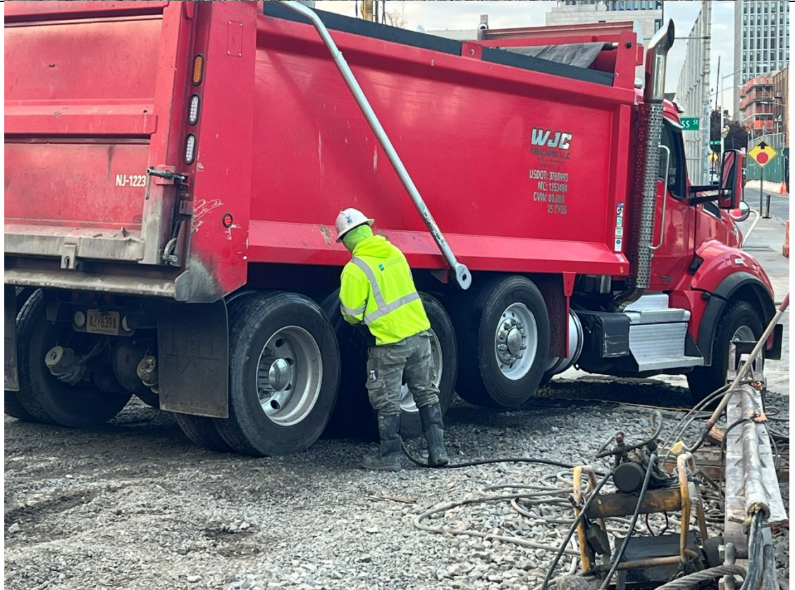
Photo 2- Representative photo of truck tire wash down.
