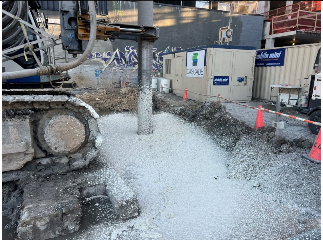
Photo 1- Representative photo of drilling an ISS column.
