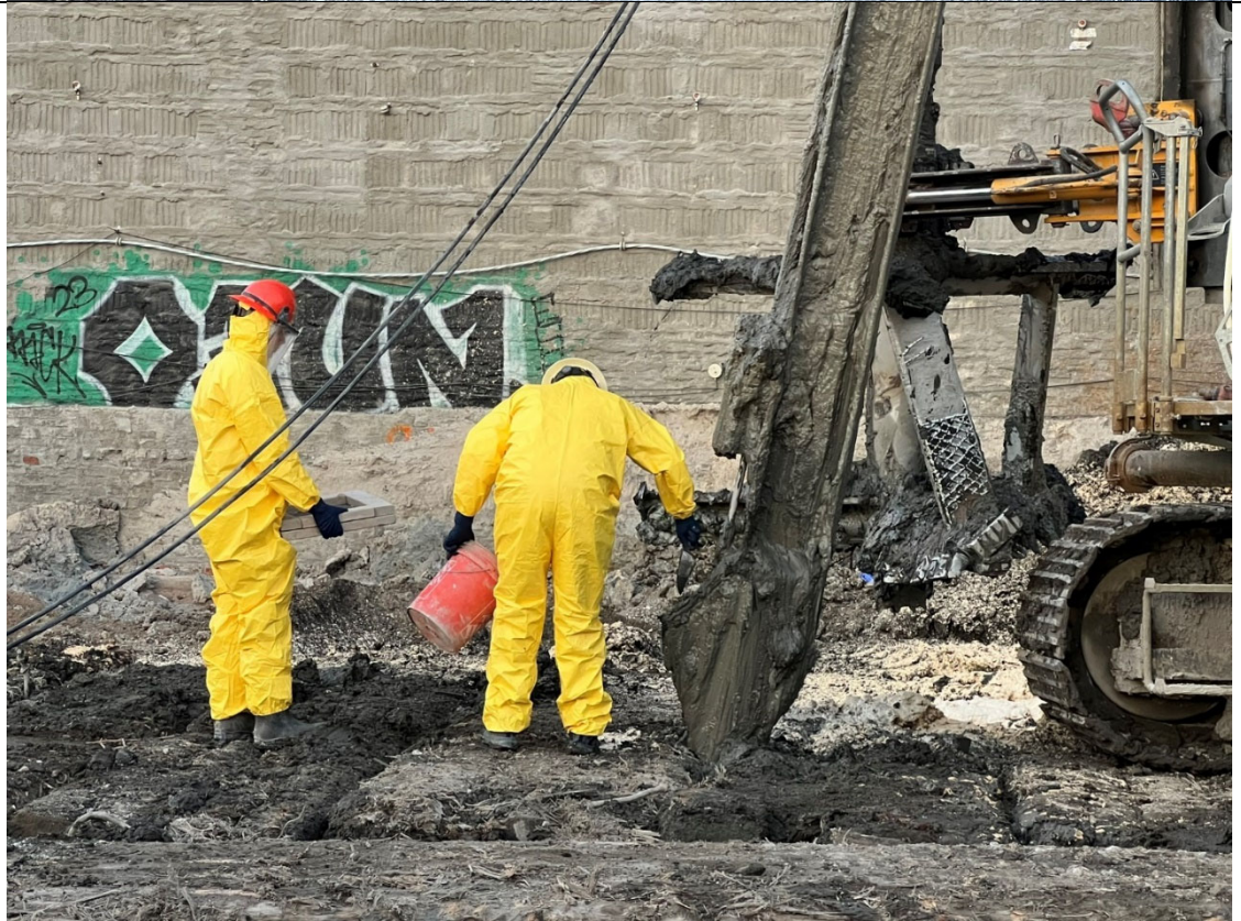
Photo 2- Representative photo of Cascade collecting a wet mix sample.
