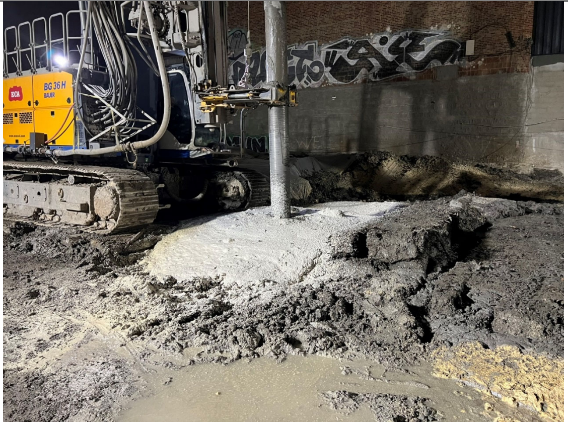
Photo 1- Representative photo of drilling an ISS column.
