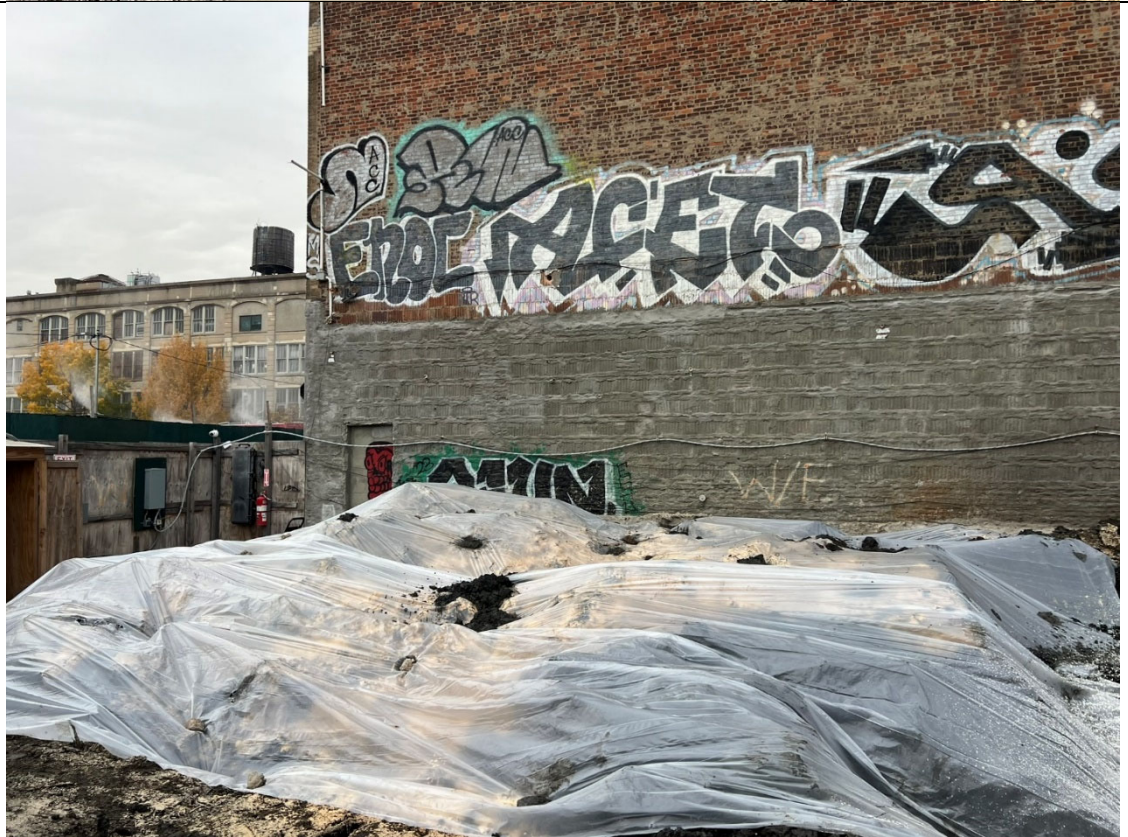
Photo 2- Representative photo of a stockpile covered with poly.
