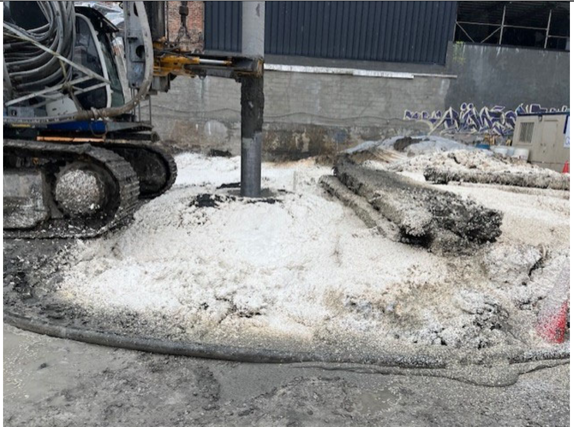
Photo 1- Representative photo of drilling an ISS column.
