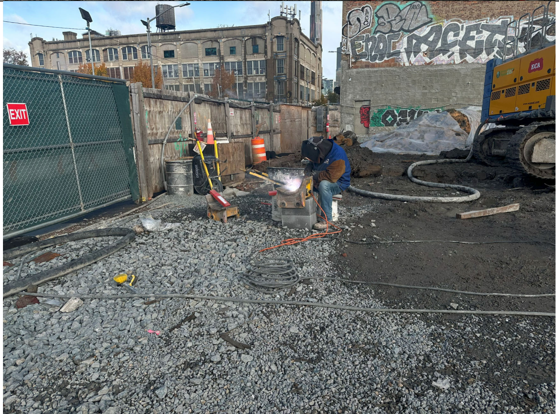
Photo 4- Additional Photo of maintenance/ welding activities.
