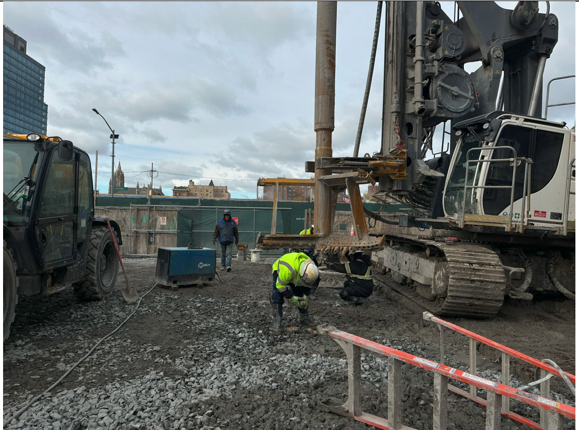
Photo 3- Representative Photo of augur maintenance.
