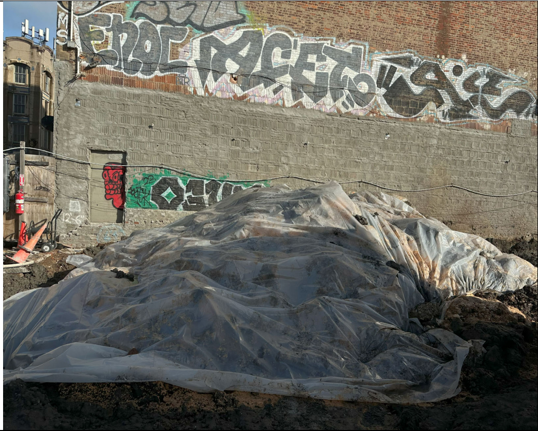
Photo 5 Representative Photo of covered stockpile.
