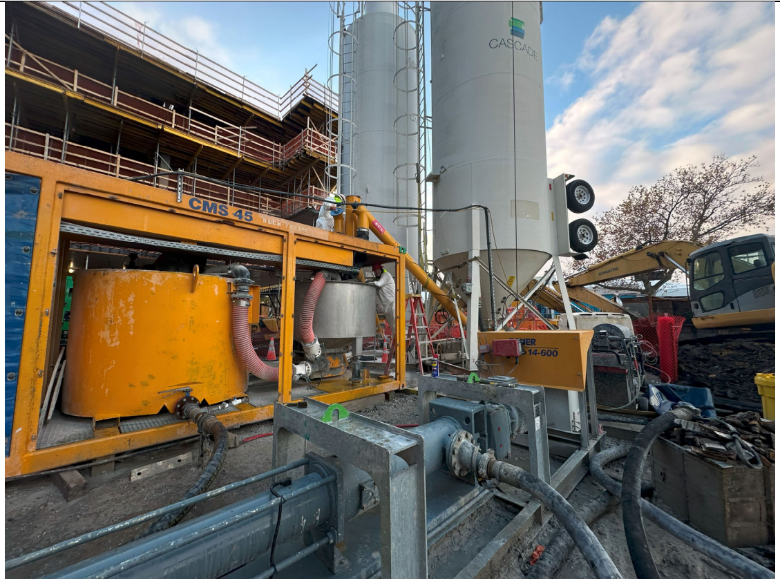
Photo 1- Representative photo of batch plant maintenance.
