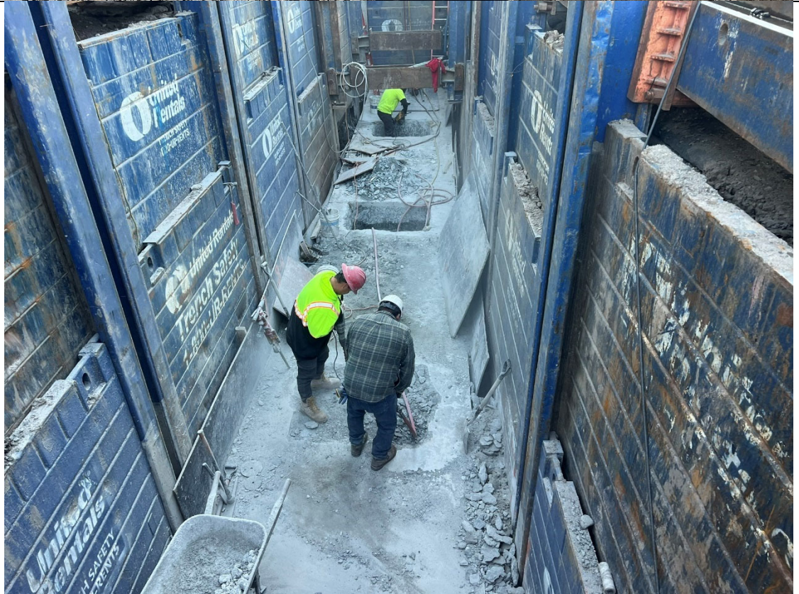
Photo 2- Representative Photo of utility vault work.
