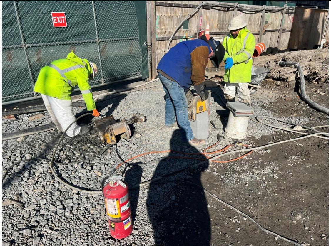
Photo 1- Representative Photo of welding and maintenance.
