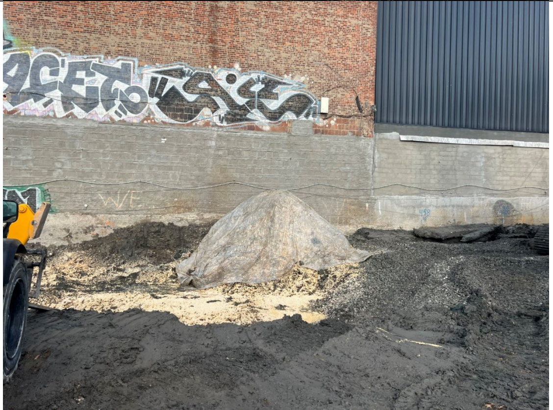
Photo 2- Representative photo of a stockpile covered with ATMOS foam and poly.
