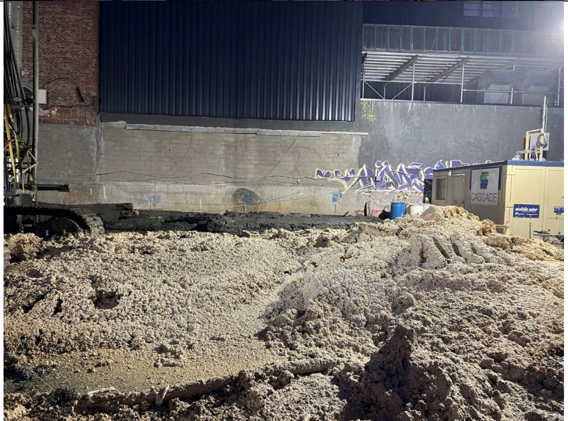
Photo 4- Representative photo of the work area sprayed with ATMOS foam at the end of the day.
