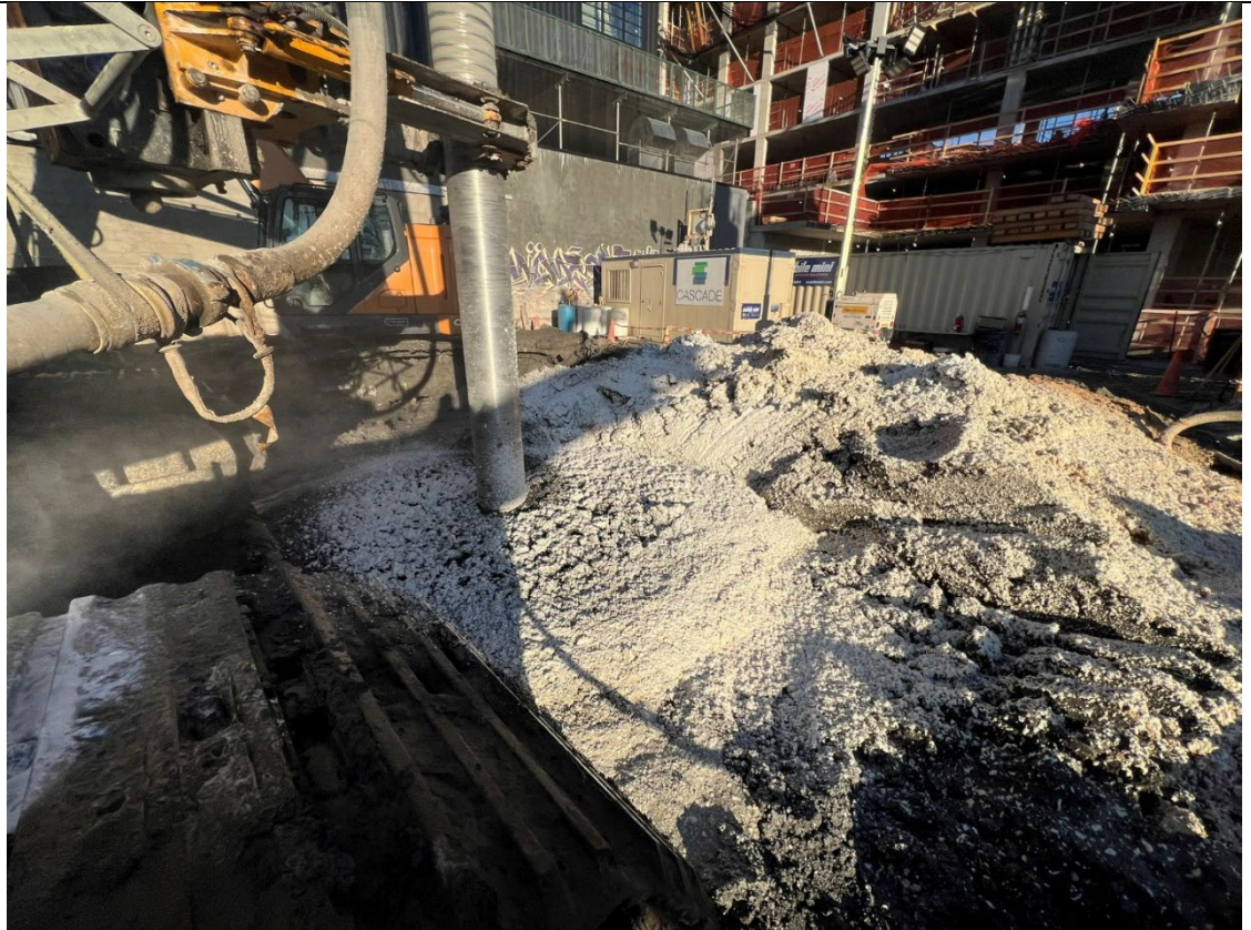
Photo 1- Representative photo of drilling an ISS column.
