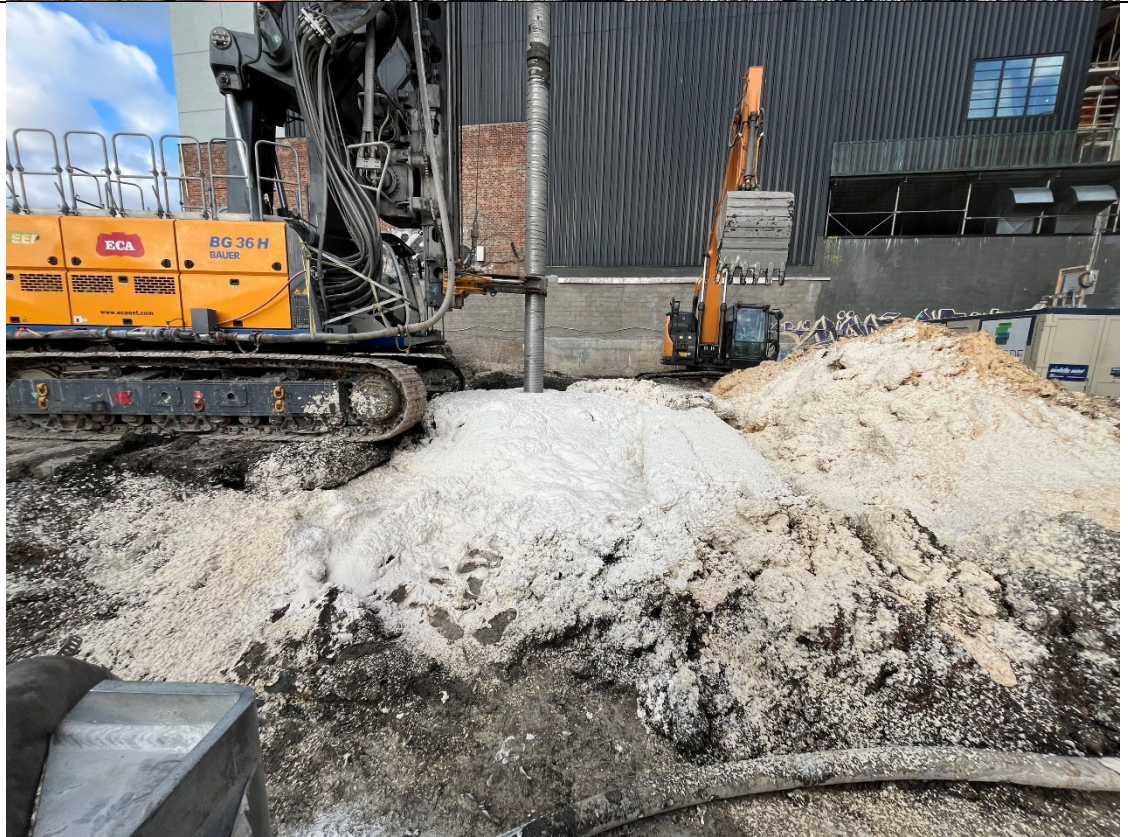
Photo 2- Representative photo of drilling an ISS column.
