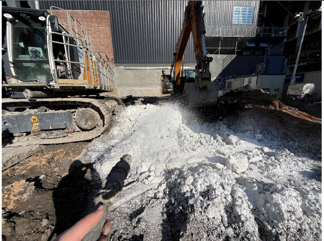
Photo 1- Representative photo of ATMOS foam application during excavation.
