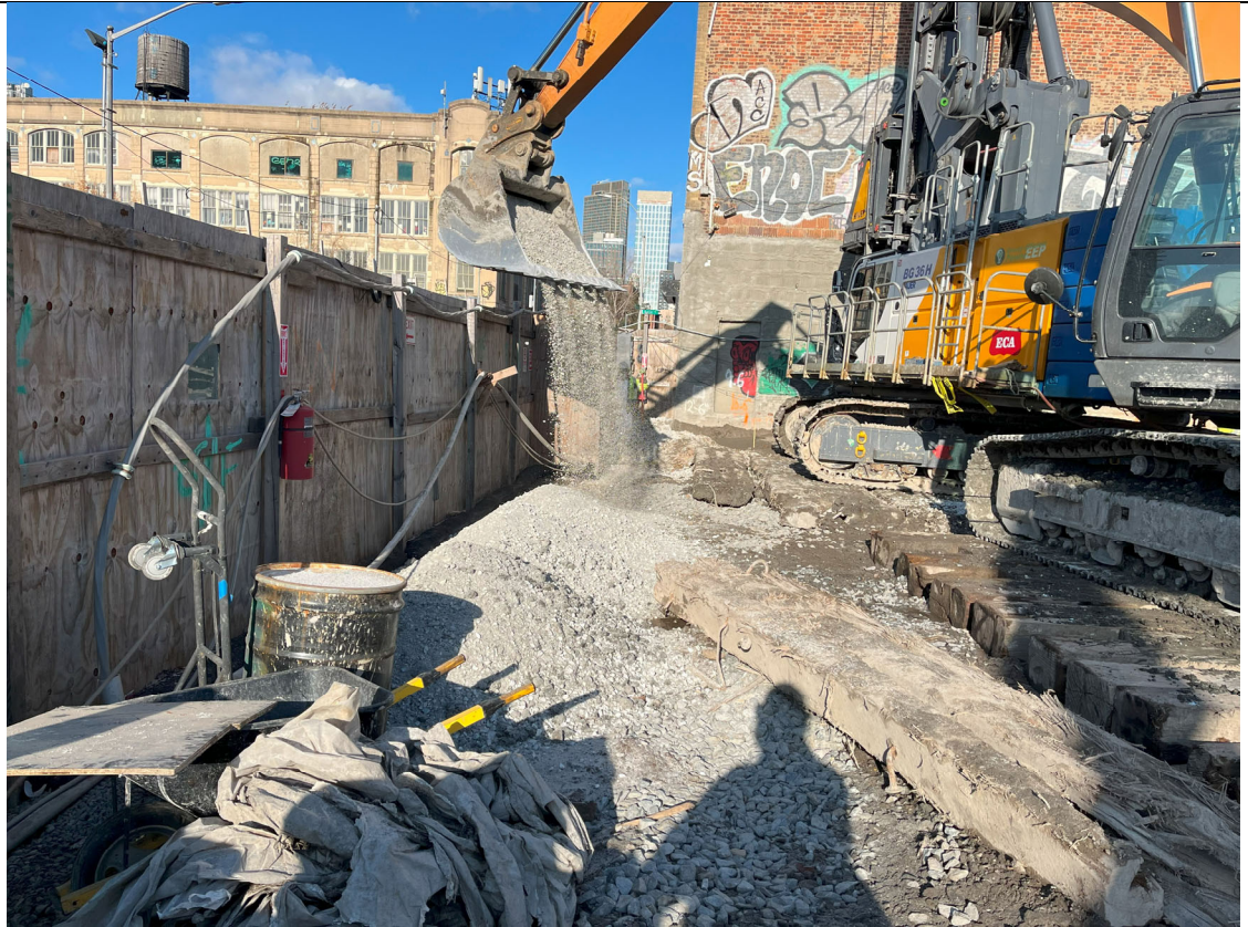
Photo 3- Representative photo of backfill delivery.
