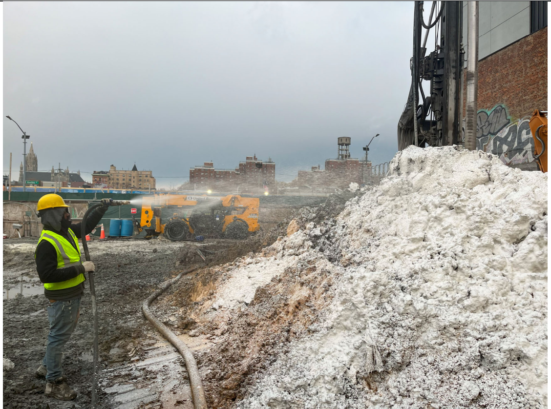
Photo 1- Representative photo of ATMOS foam application.
