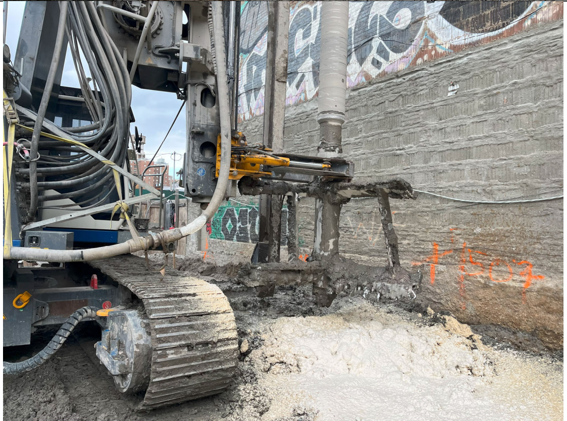
Photo 2- Representative photo of ISS installation.
