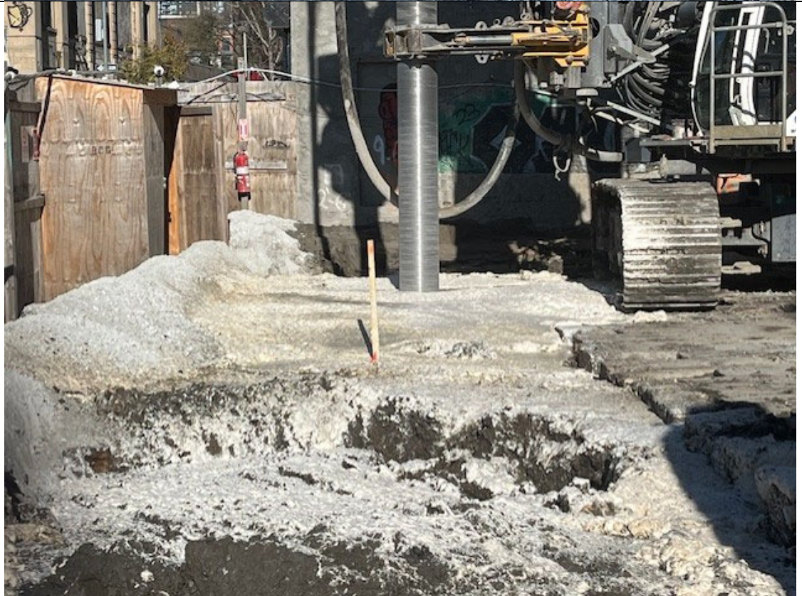
Photo 2- Representative photo of ISS installation.
