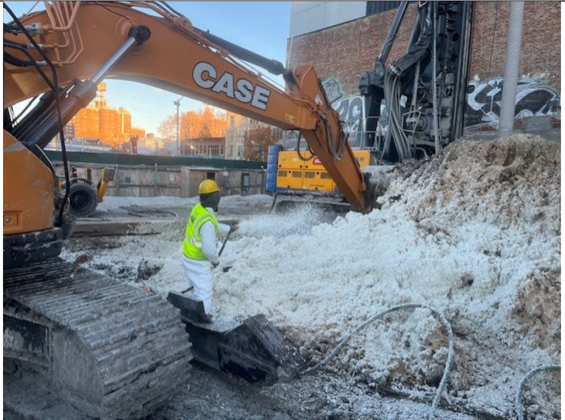
Photo 1- Representative photo of ATMOS foam application on swell stockpile during trucking events.
