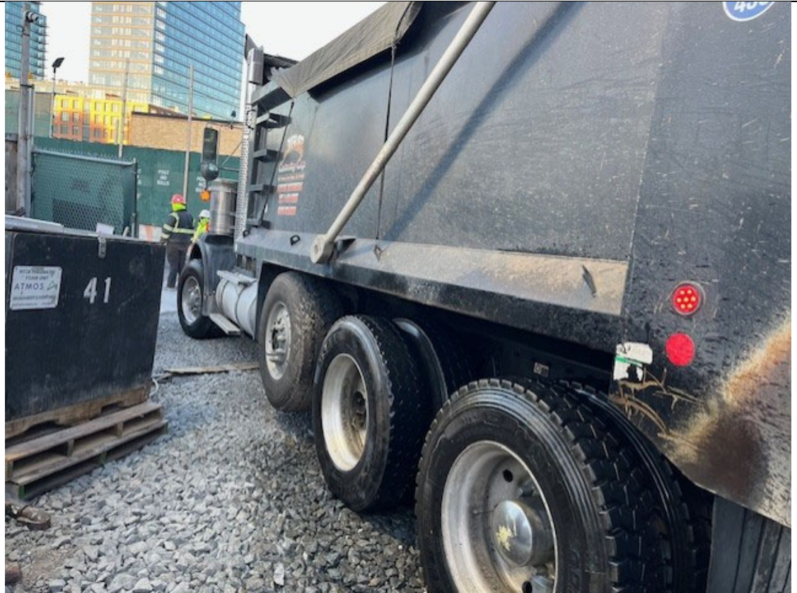
Photo 3- Representative photo of backfill delivery.
