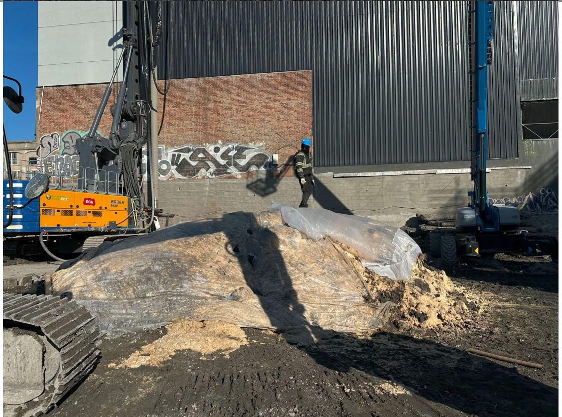
Photo 4- Additional Photo of the swell stockpile being covered in poly at the end of activities.
