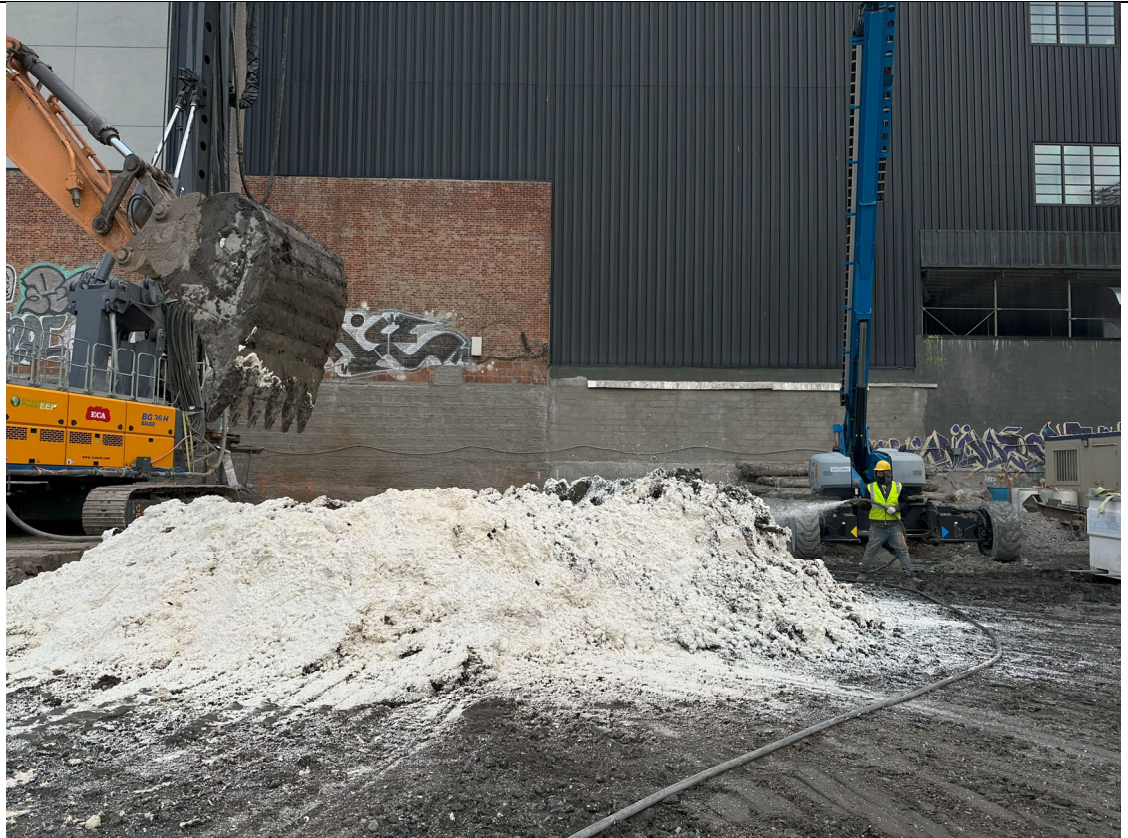
Photo 3- Representative Photo of Atmos foam application to swell stockpile.
