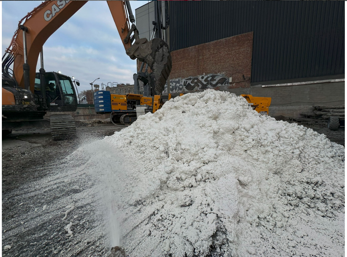
Photo 2- Representative photo Atmos foam being applied as swell material being moved.
