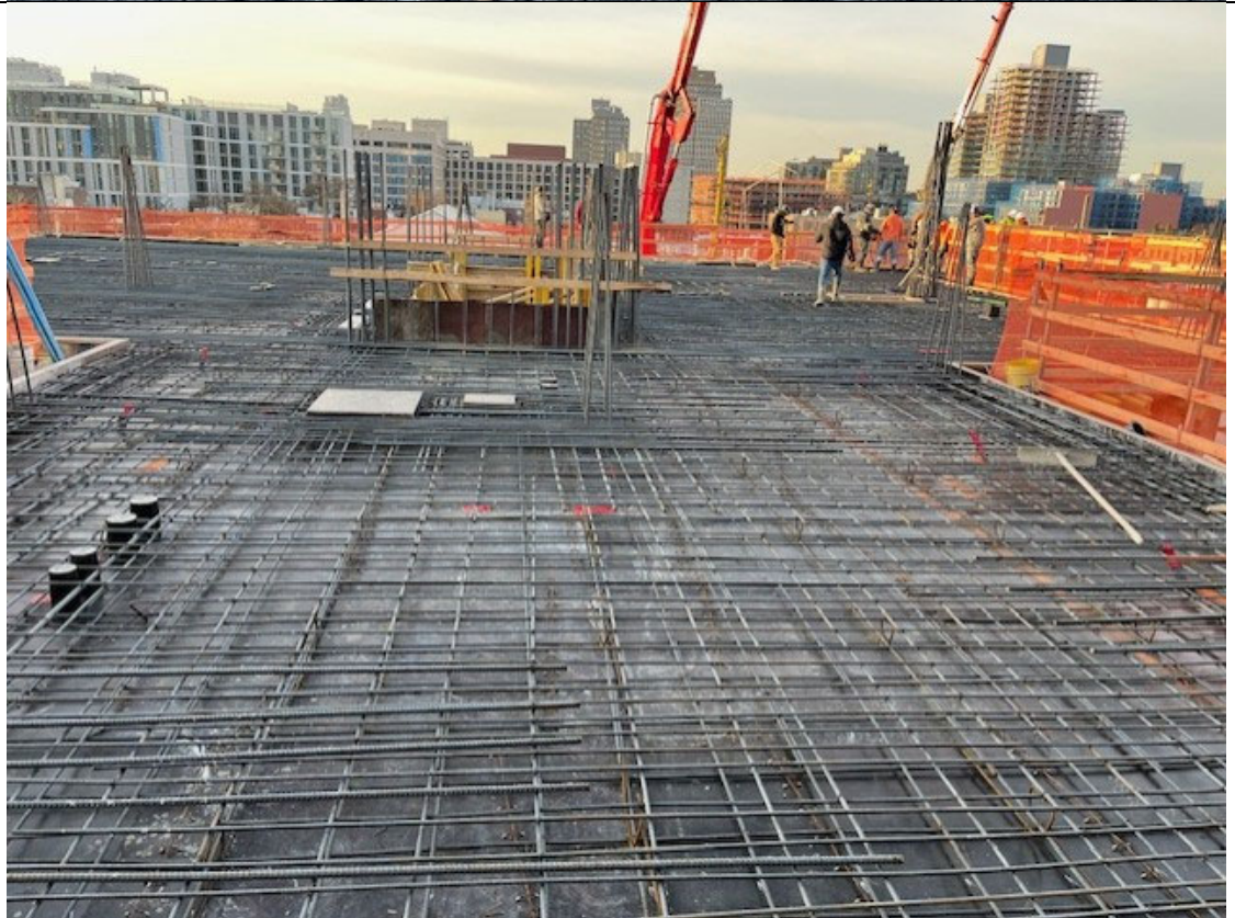
Photo 4- Representative photo of slab- on-deck concrete placement.
