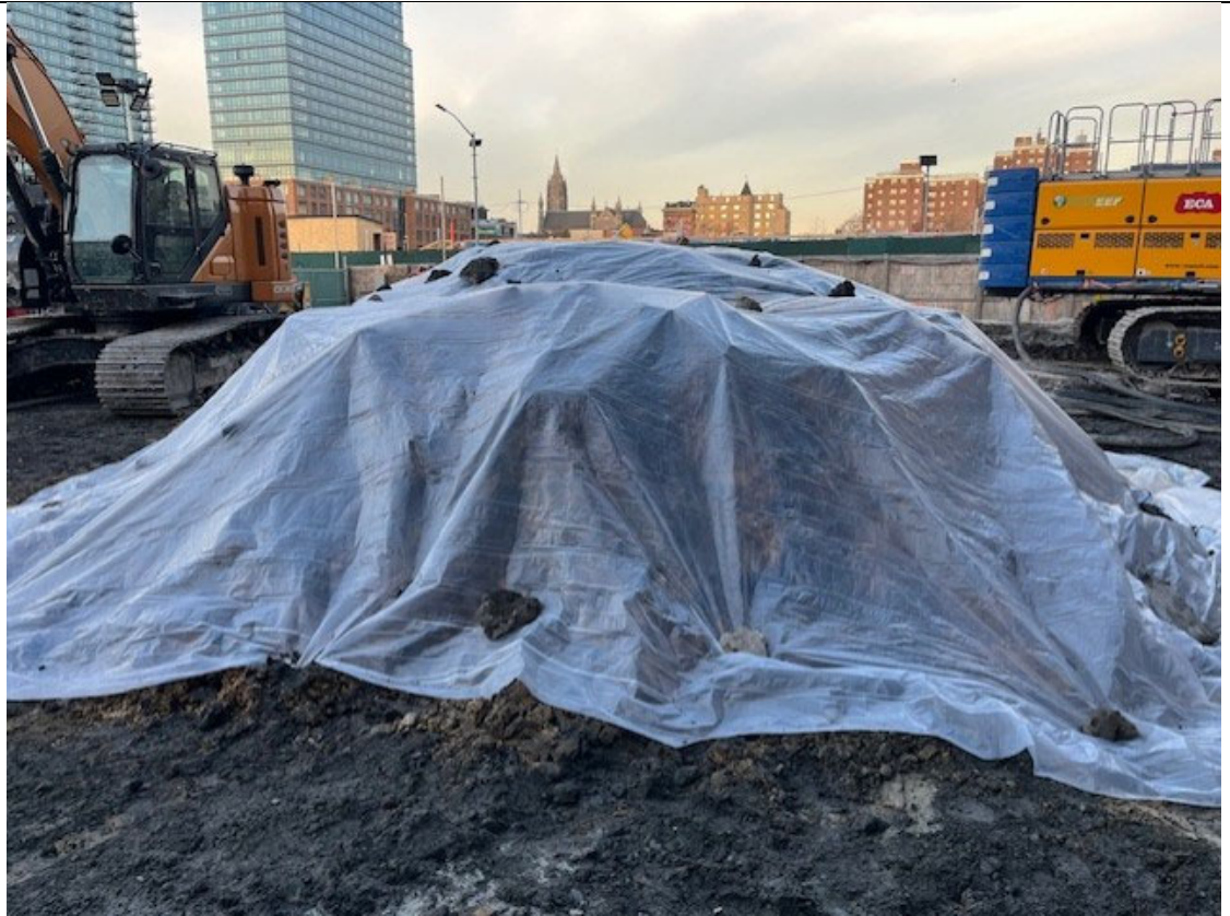
Photo 3- Representative photo of stockpile covered with Poly.
