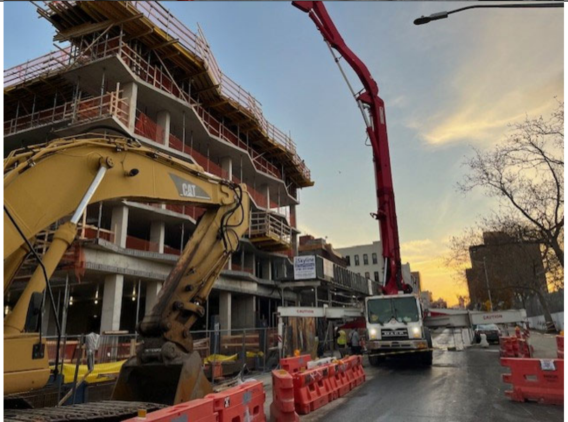
Photo 2- Representative photo of concrete pump setup.
