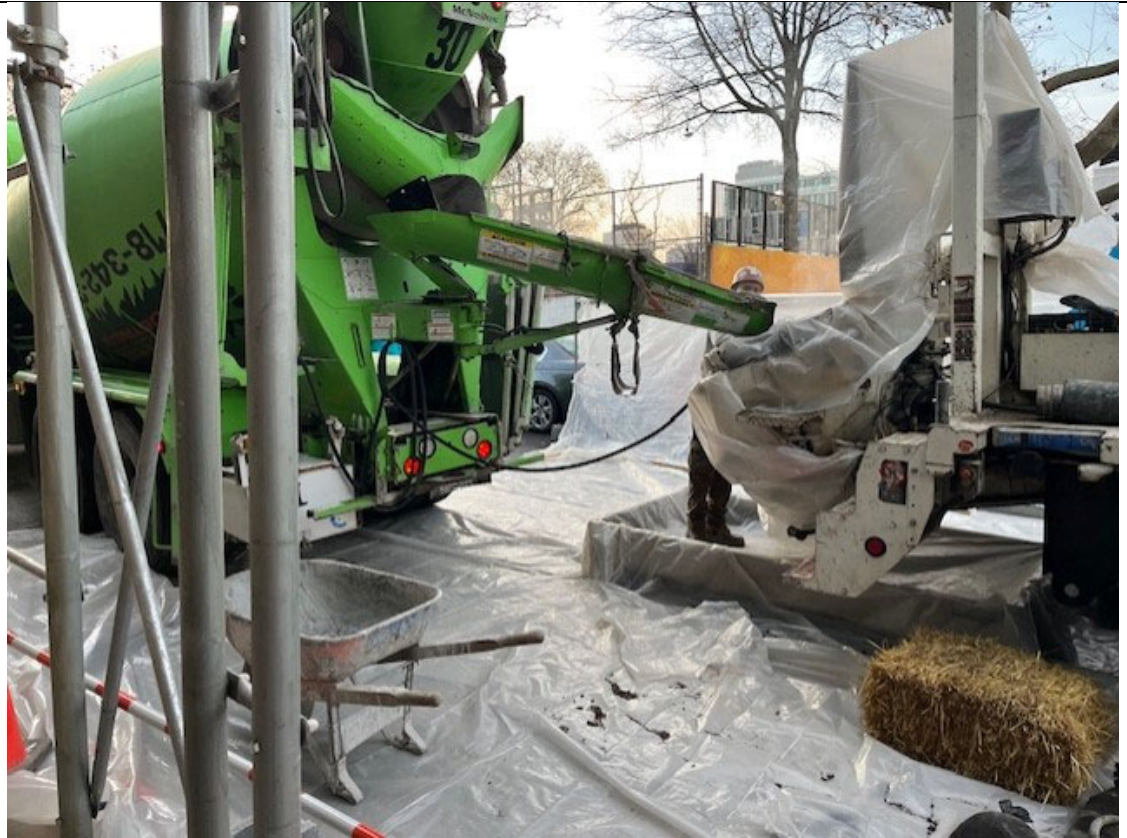
Photo 1- Representative photo of concrete area placement.
