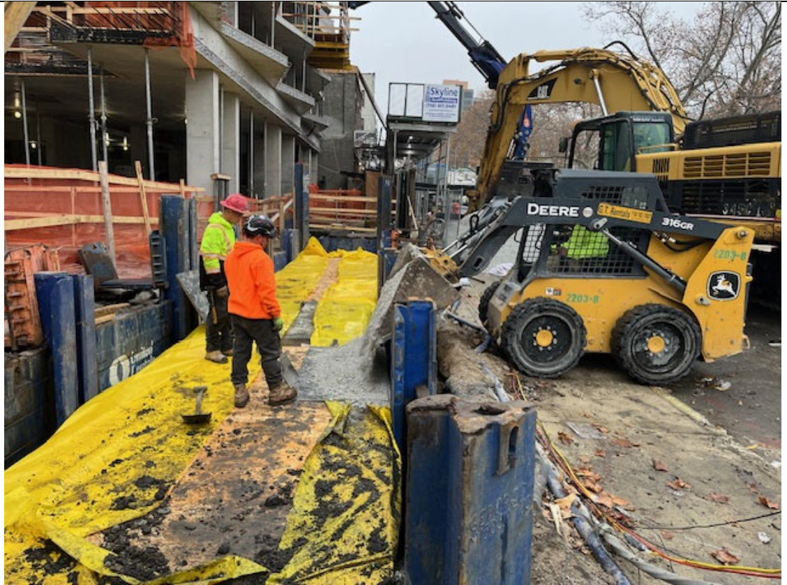
Photo 3- Representative photo of backfilling Con Ed Vault.
