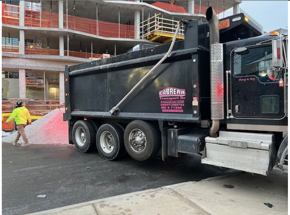
Photo 1- Representative photo of DGABC Limestone delivery for Con Ed Vault.
