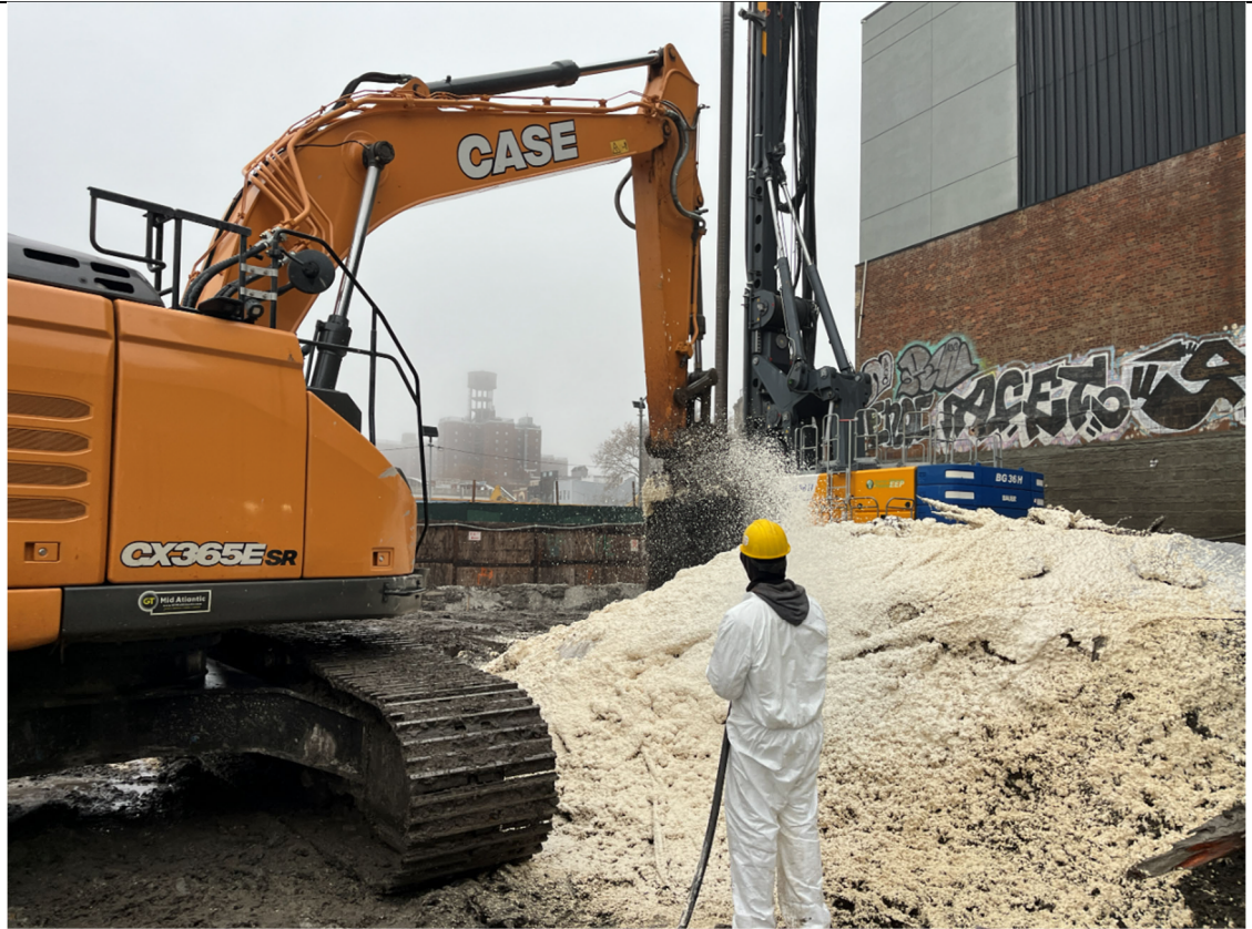
Photo 1- Representative photo of ATMOS foam application during swell material loadout.
