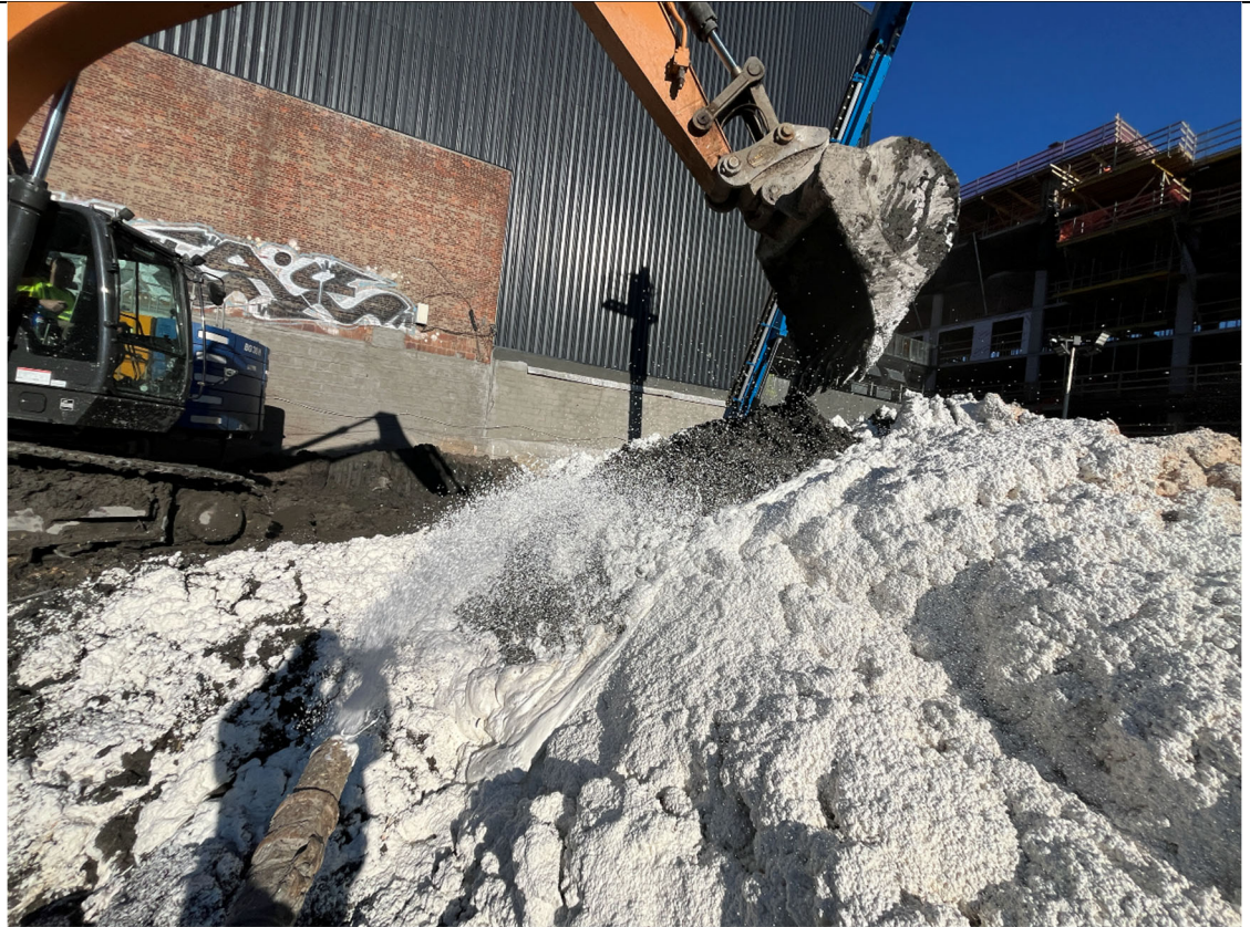
Photo 1- Representative photo of ATMOS foam application.
