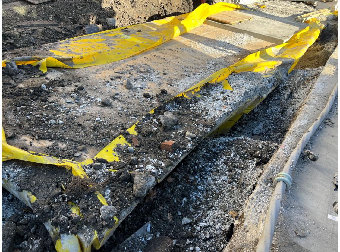
Photo 3- Representative photo of backfilled utility vault.
