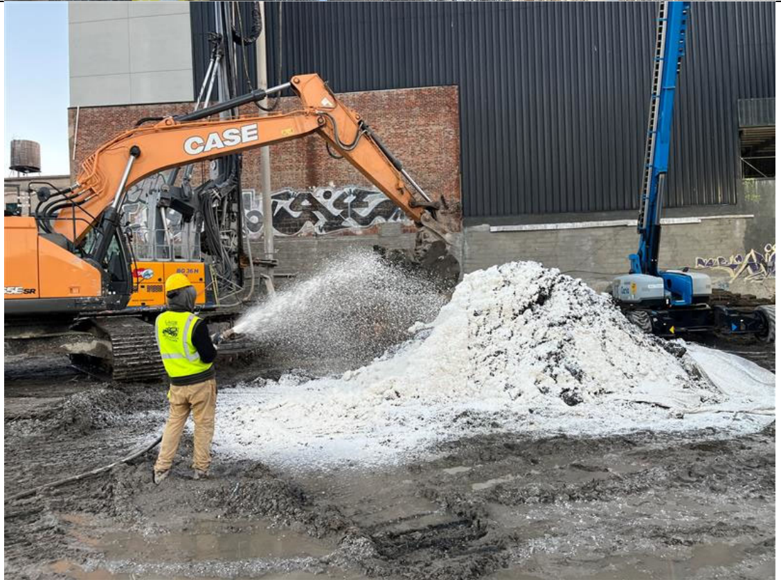
Photo 4- Representative photo of ISS application to stockpile.
