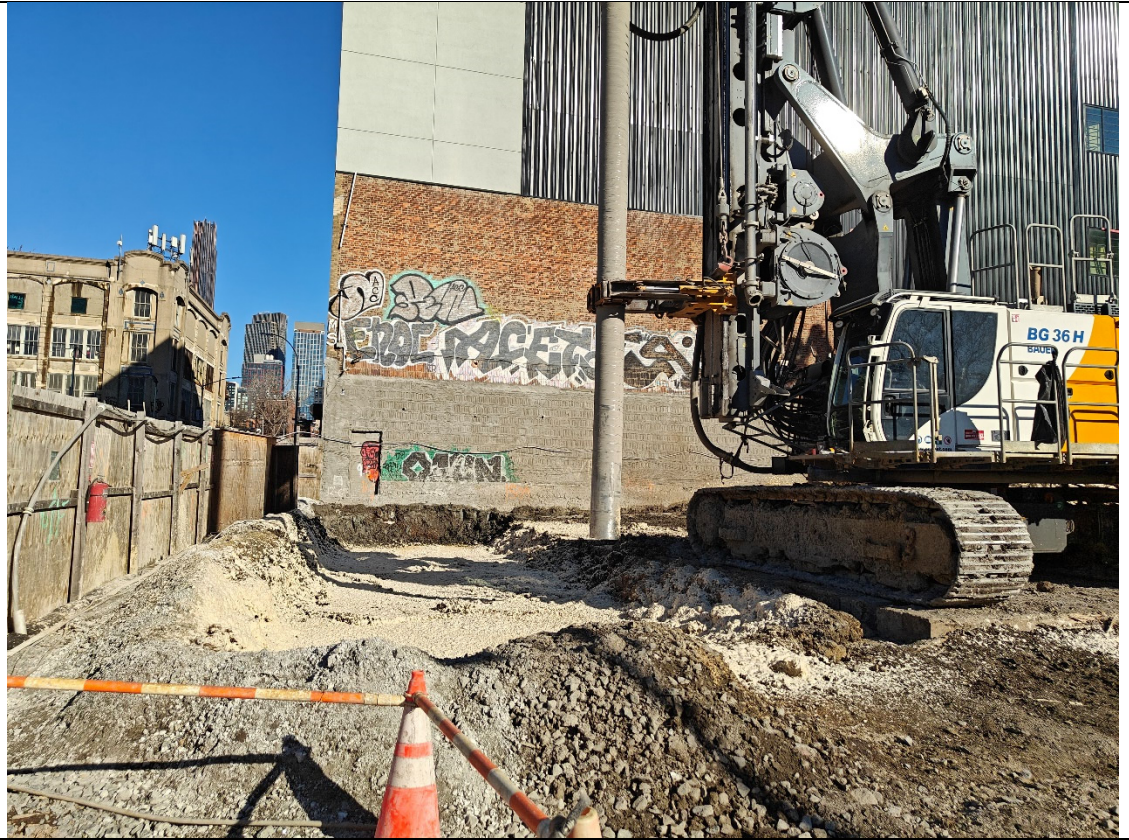
Photo 3- Representative photo of ATMOS applied to swell excavation area.
