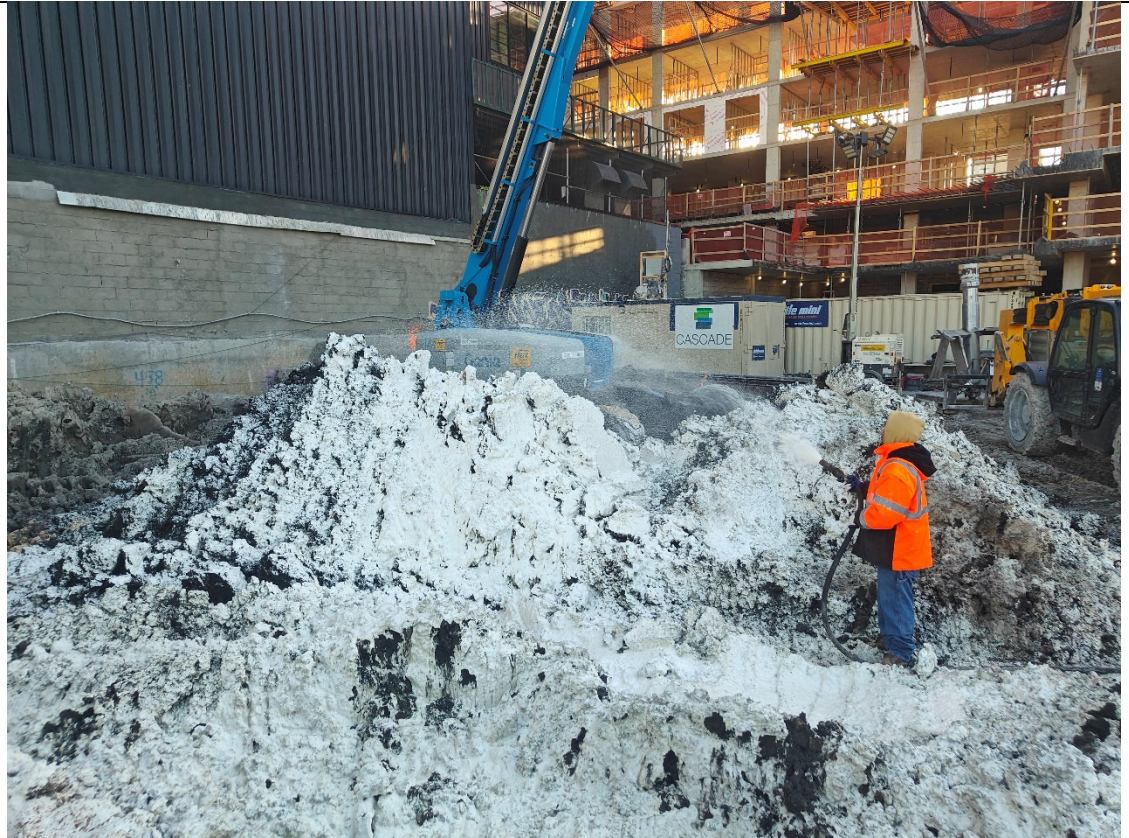
Photo 1- Representative photo of ATMOS foam application.
