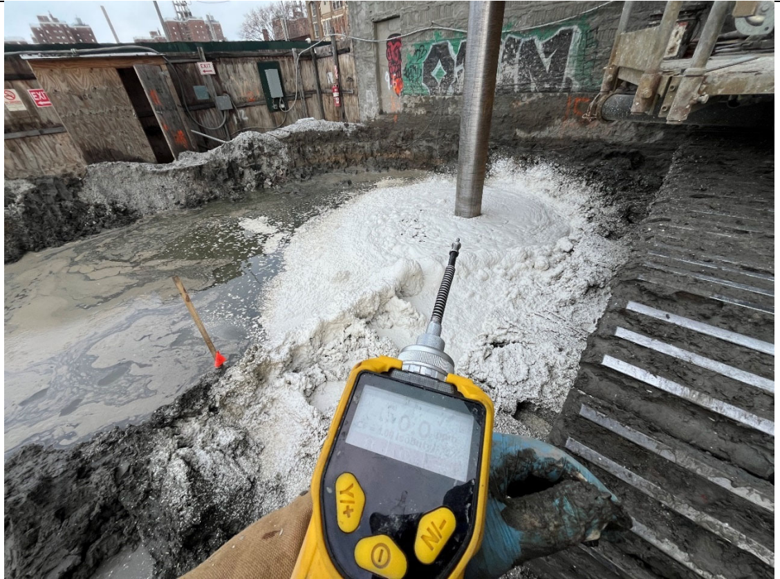
Photo 1- Representative photo of ISS column installation.
