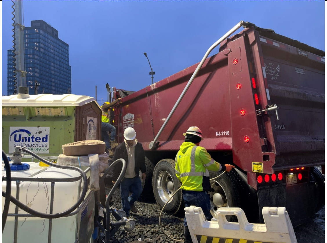
Photo 4- Representative photo of truck tires being washed and cover strapped down securely.
