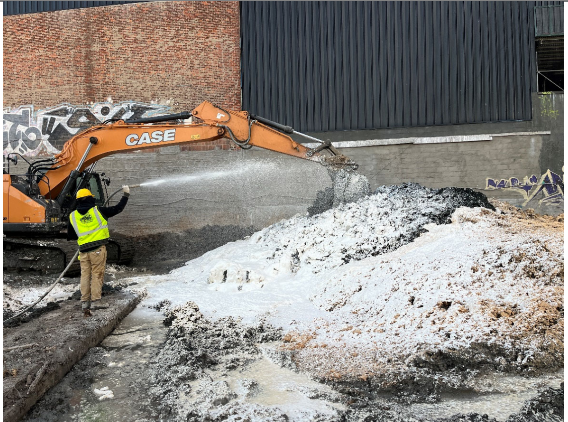
Photo 3- Representative photo of ATMOS foam applied to Swell Stockpile area.
