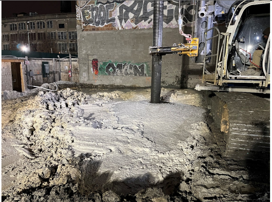
Photo 1- Representative photo of ISS column installation.
