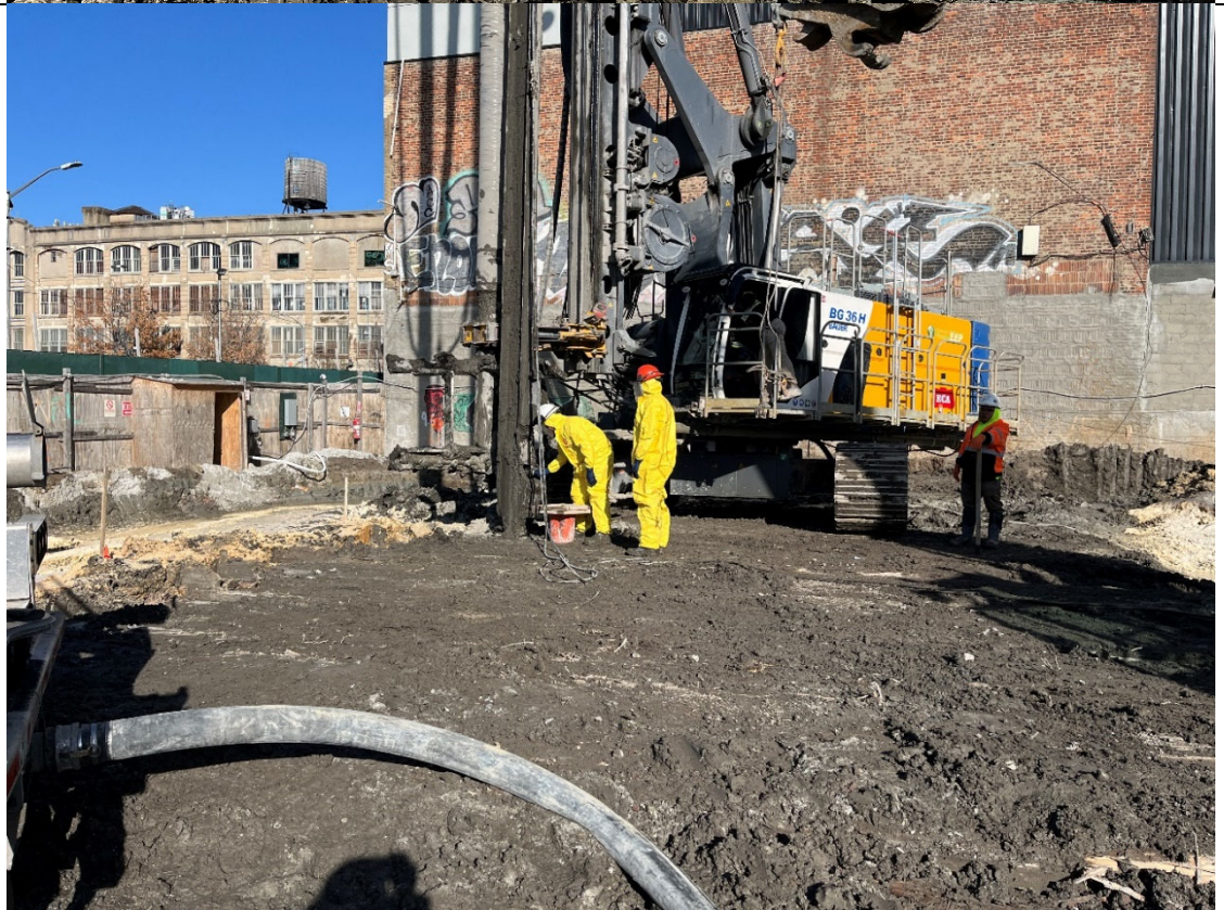
Photo 2- Representative photo of wet mix sampled on column 381.
