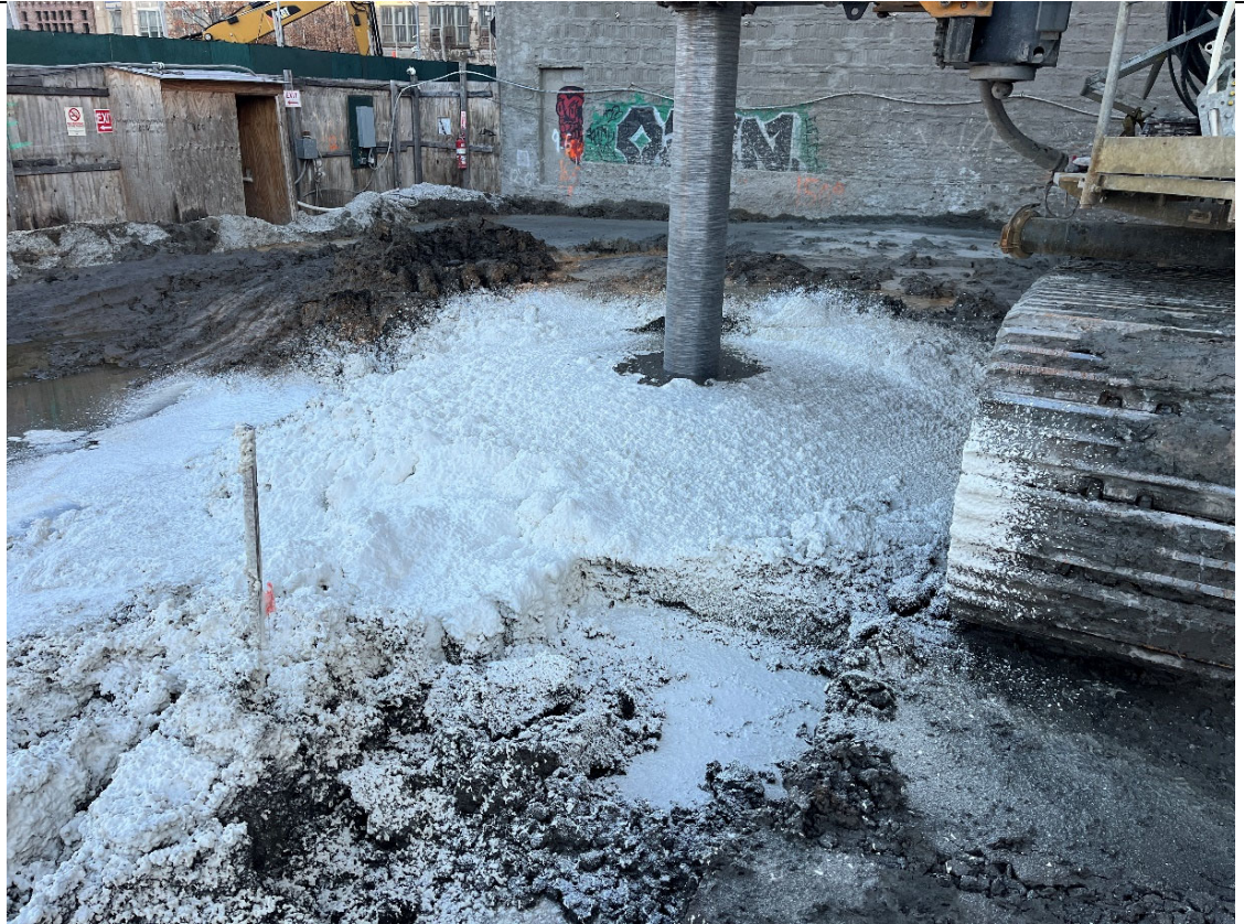
Photo 1- Representative photo of ISS column installation.
