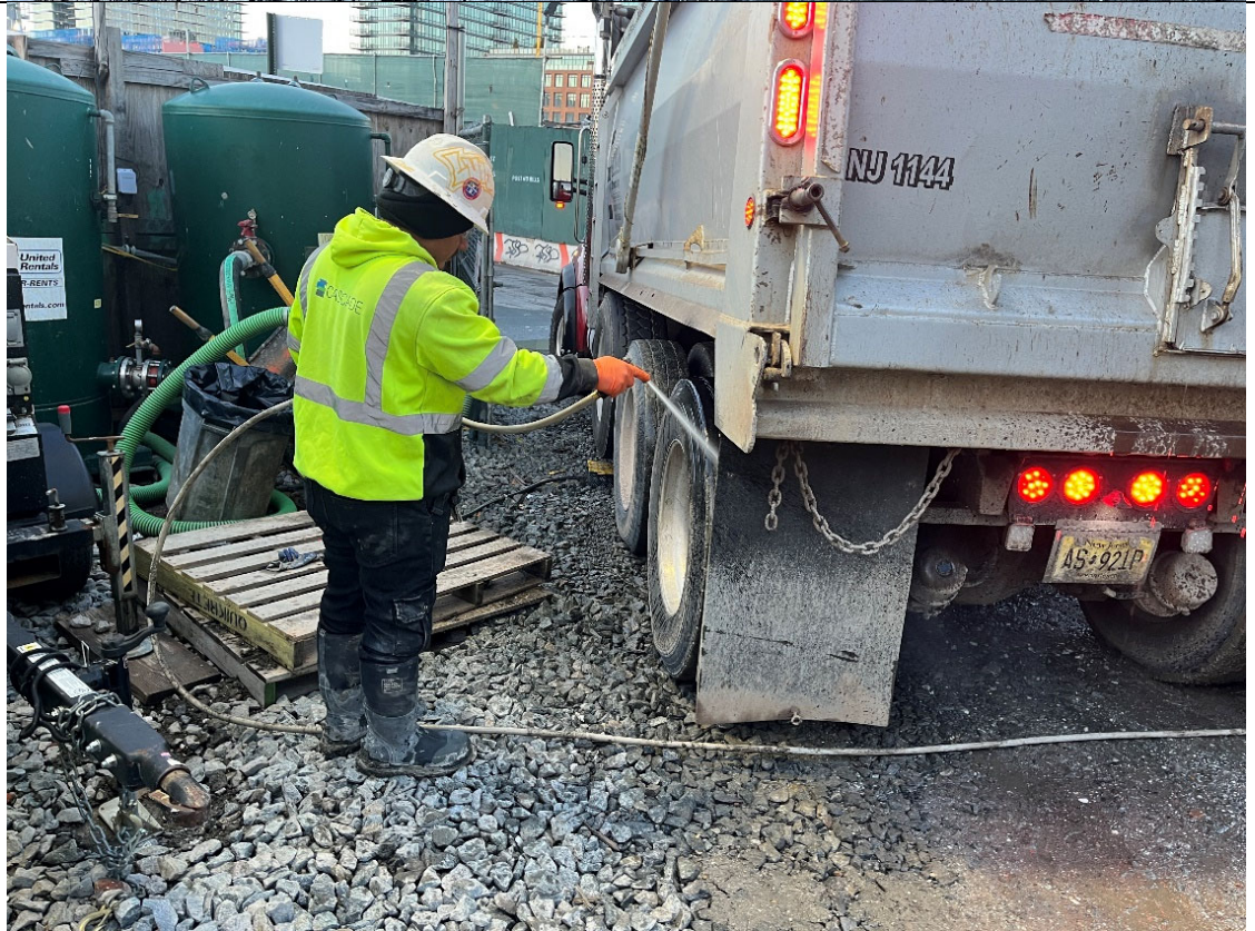
Photo 2- Representative photo of trucks tires being washed before leaving the site.
