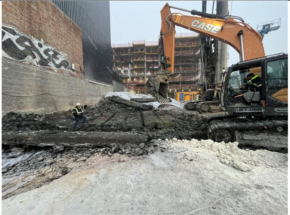
Photo 3- Representative photo of relocating drilling mats.
