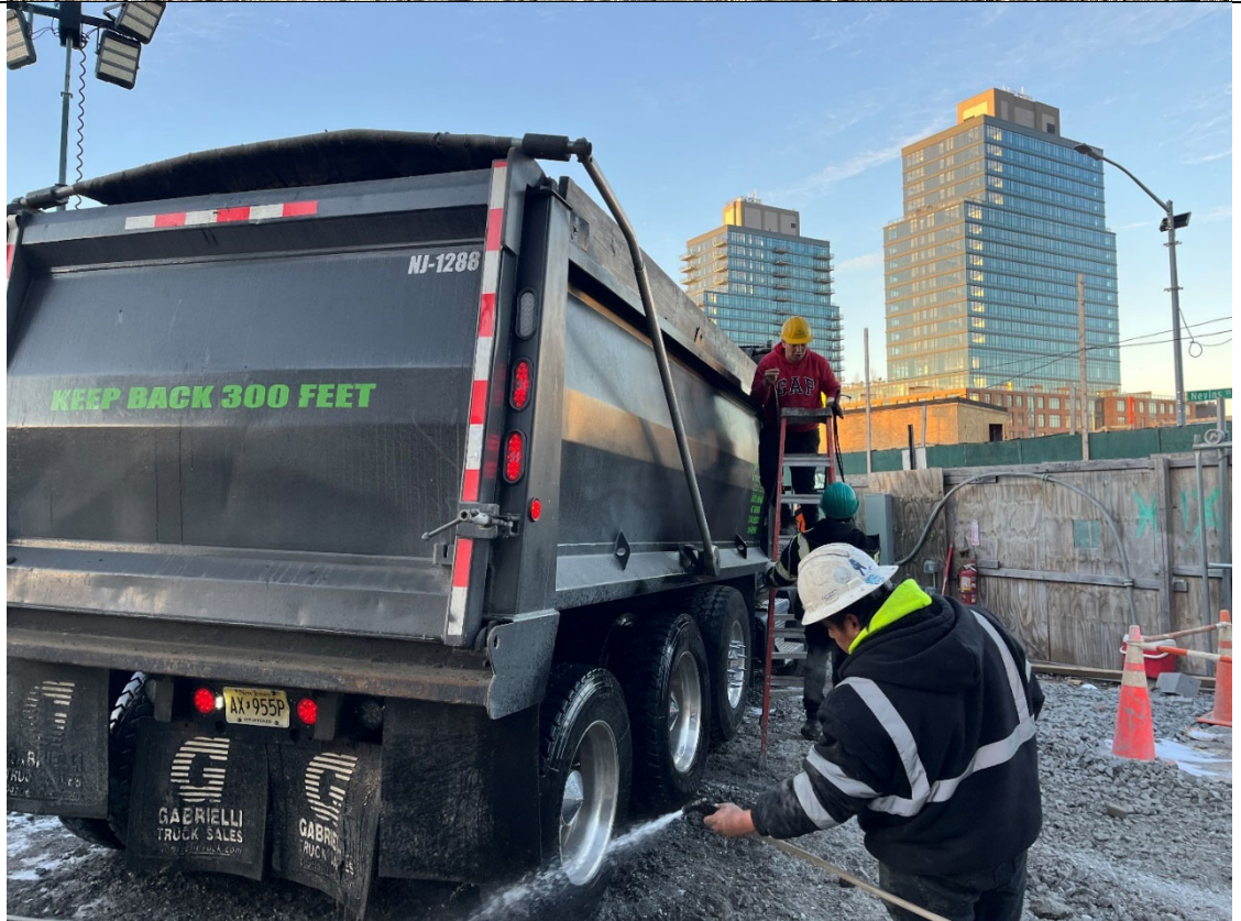
Photo 2- Representative photo of washing wheels and straps placed before truck leaves site.
