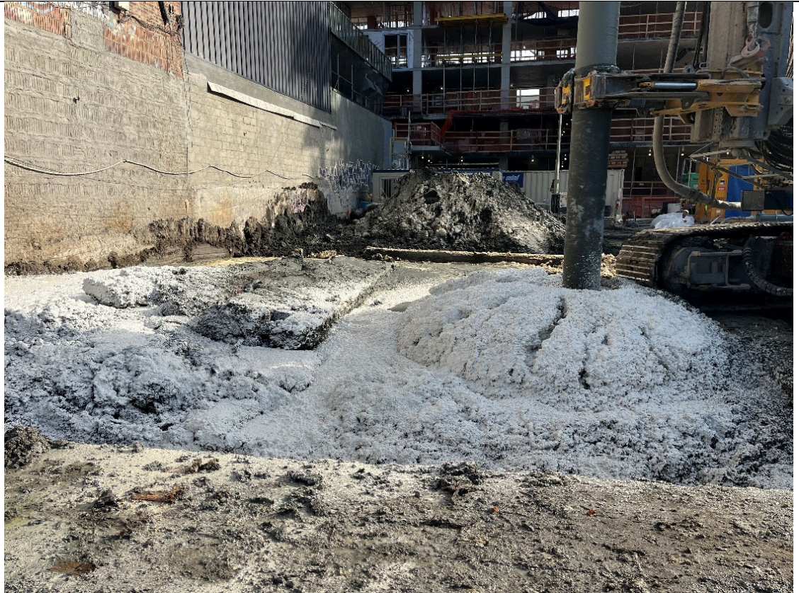
Photo 1- Representative photo of ISS column installation.
