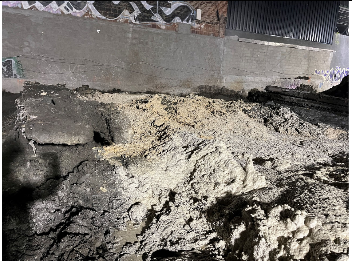
Photo 3- Representative photo of ISS column installation area at end of day.
