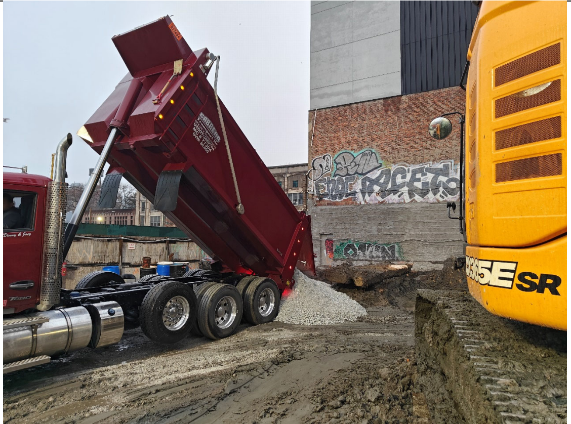
Photo 3- Representative photo of backfill delivery.
