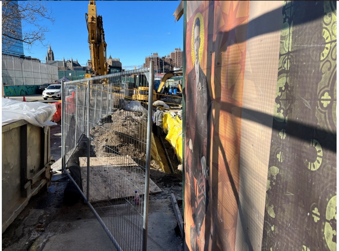
Photo 4- Representative photo utility vault work.
