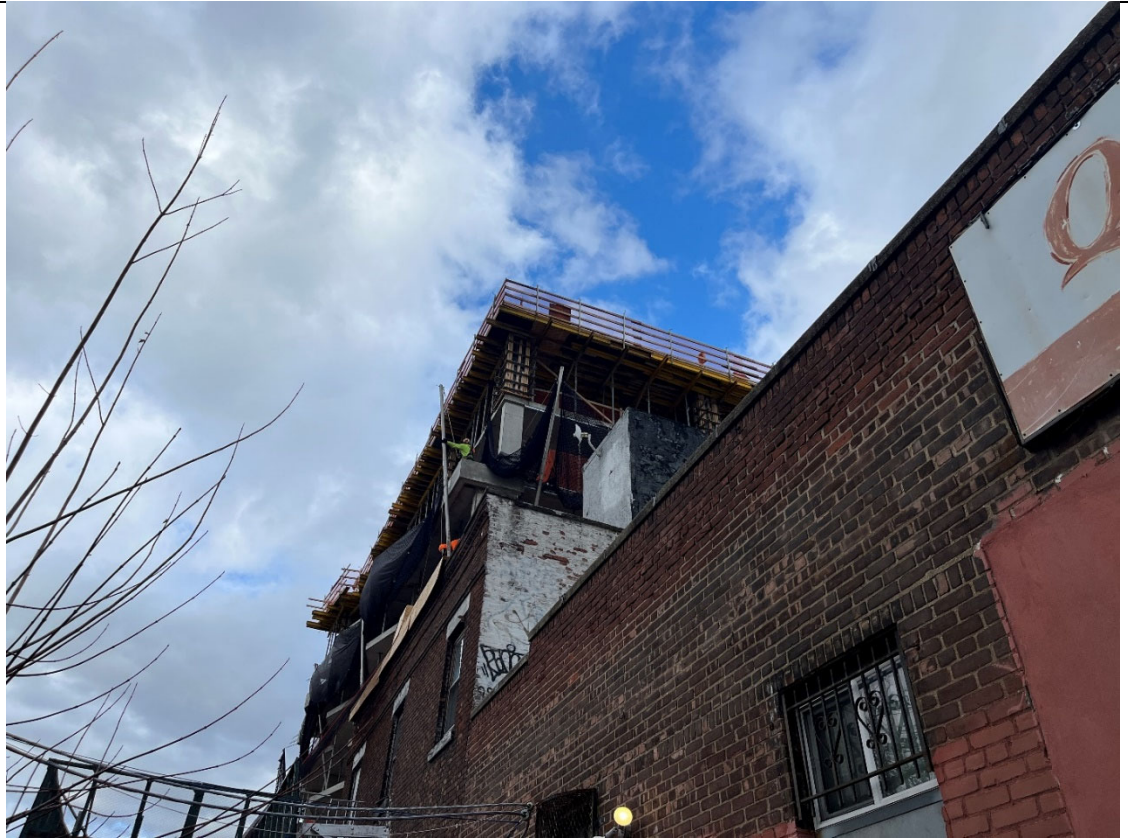
Photo 3- Representative photo of superstructure work.
