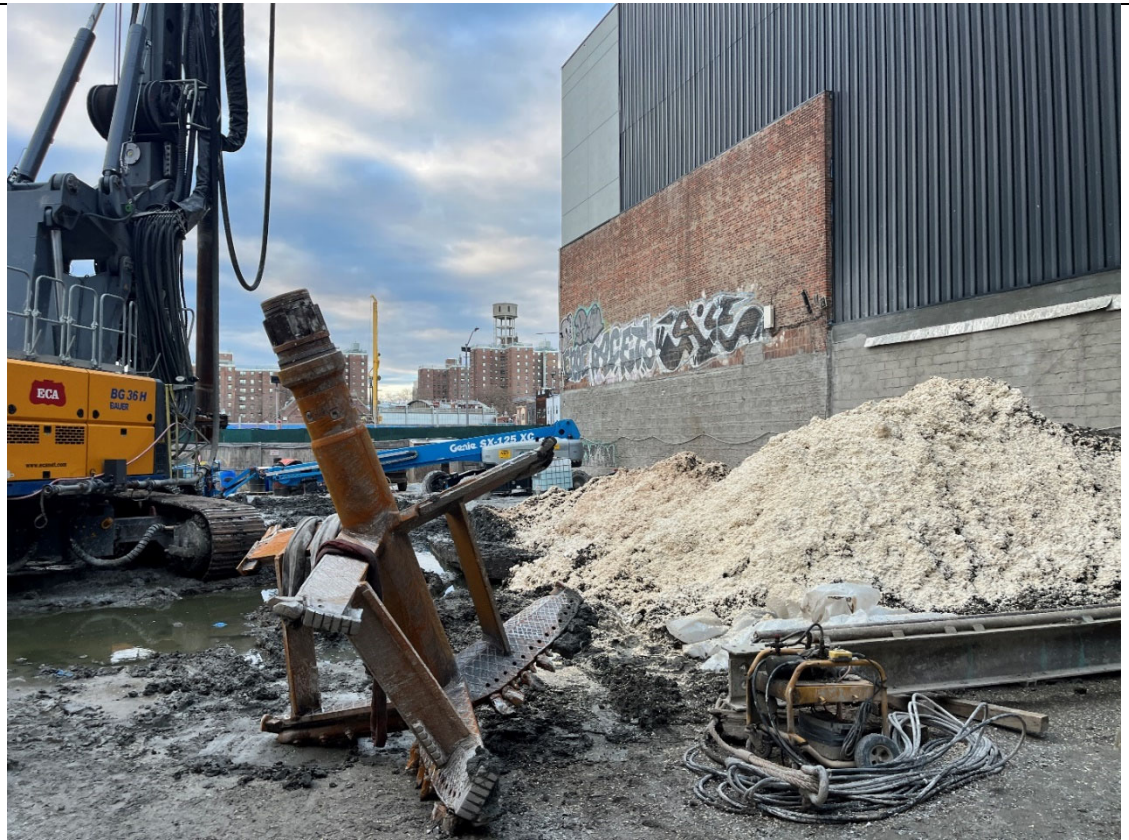
Photo 5- Representative photo of the ISS auger and the swell stockpile covered with Atmos foam.
