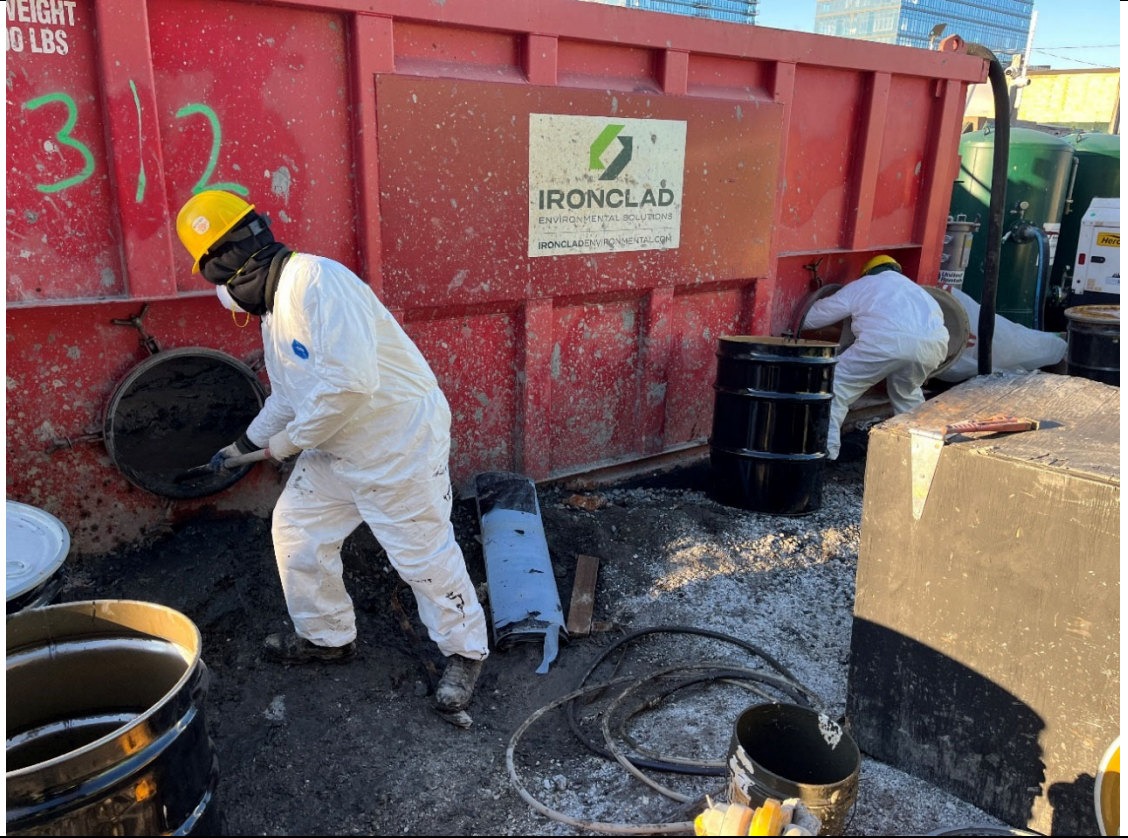
Photo 2- Representative photo of containerizing sediment from frac tank.
