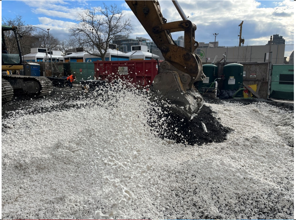
Photo 1- Representative photo of applying Atmos foam to excavation area.
