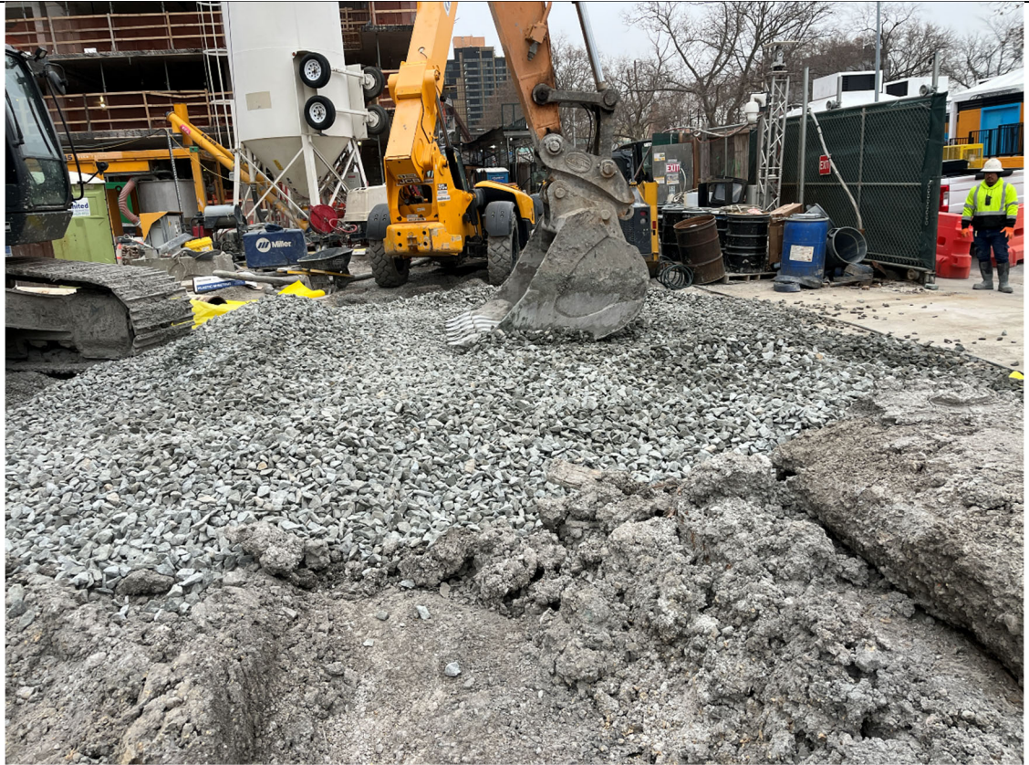
Photo 1- Representative photo of trucking pad construction.
