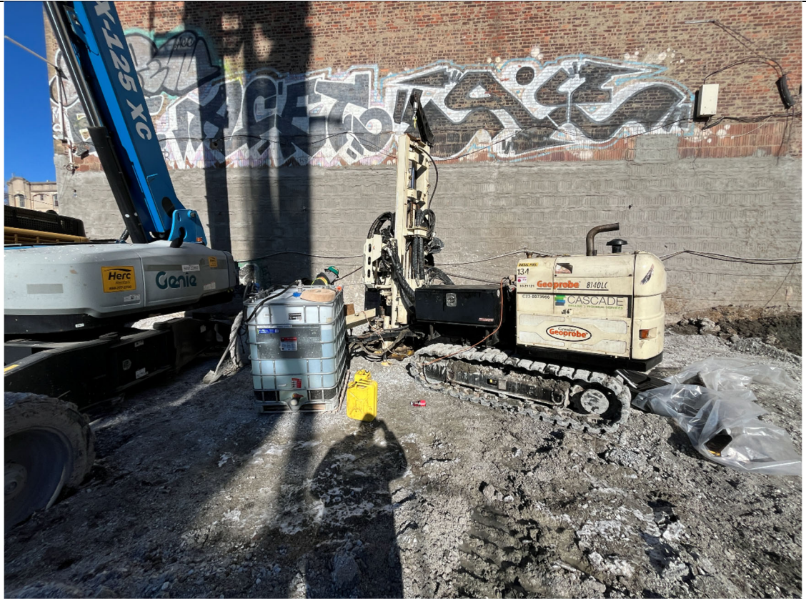
Photo 1- Representative photo ISS Core drilling.
