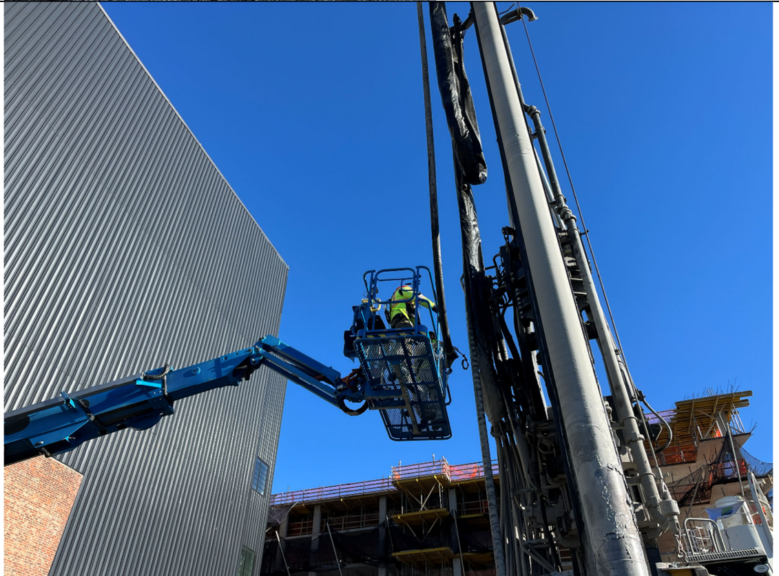
Photo 4- Representative photo of rig maintenance.
