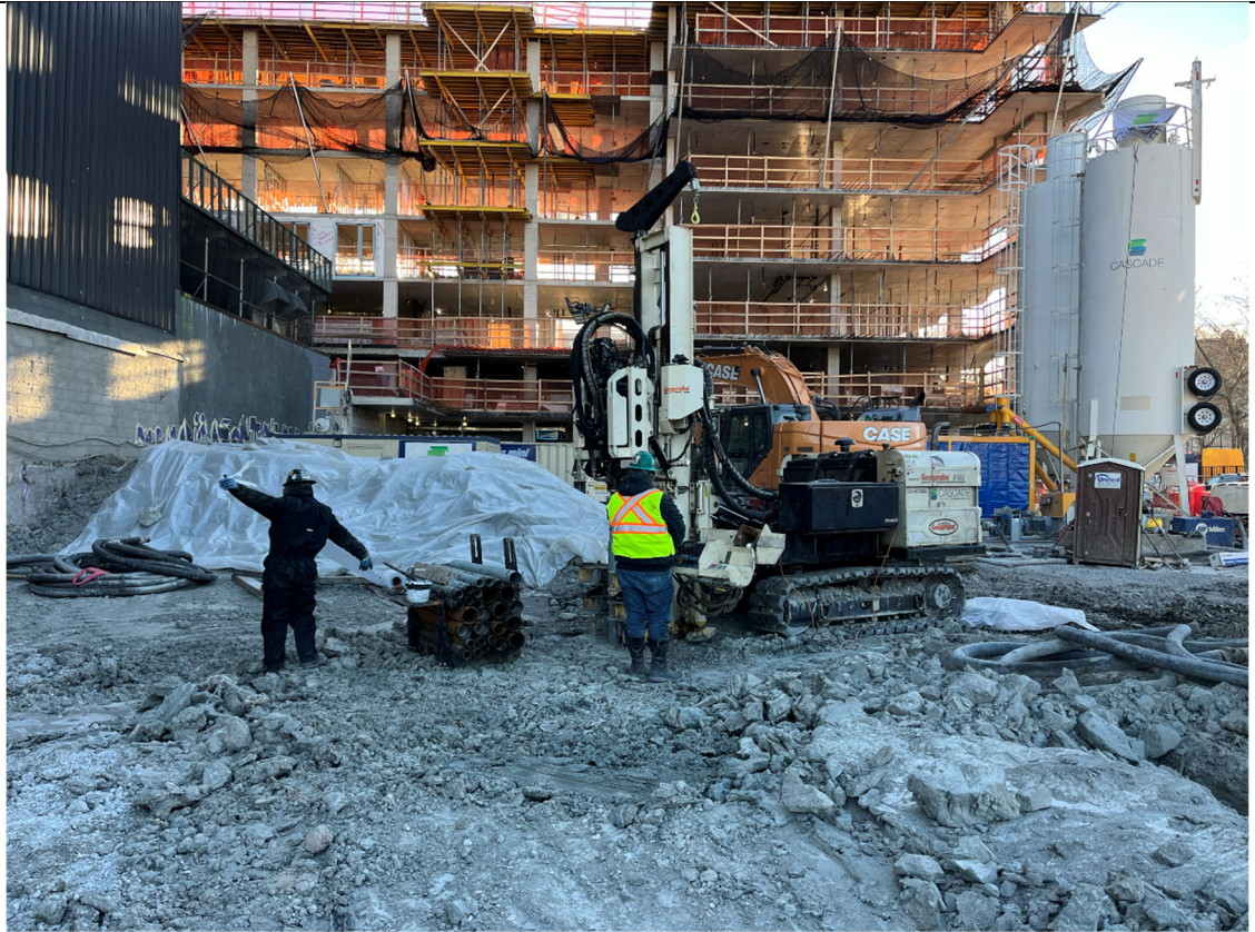
Photo 1- Representative photo ISS Core drilling.
