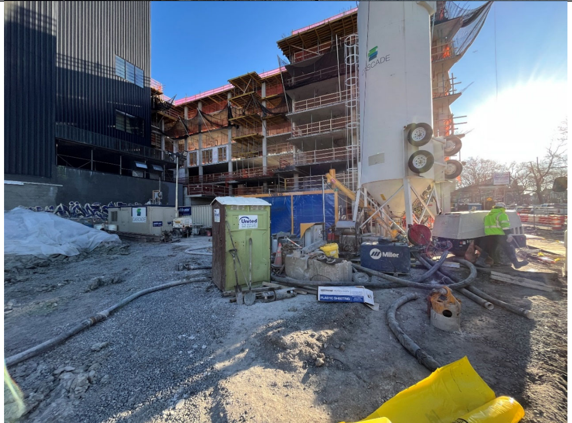
Photo 4- Representative photo of superstructure.
