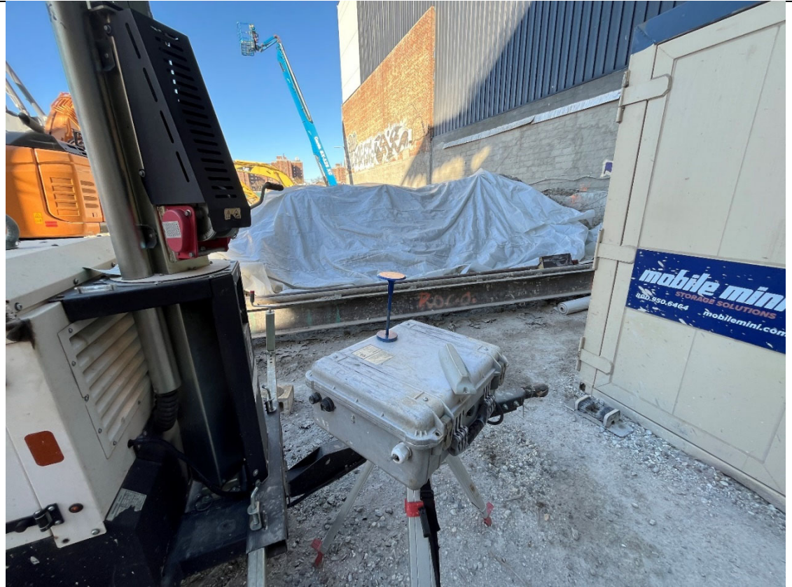
Photo 3- Representative photo of ISS Stockpile covered with poly.
