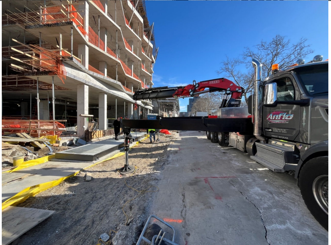
Photo 2- Representative photo of utility vault top delivery.
