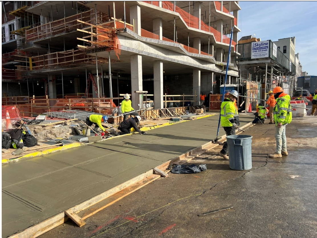
Photo 1- Representative photo of con ed vault concrete finishing.
