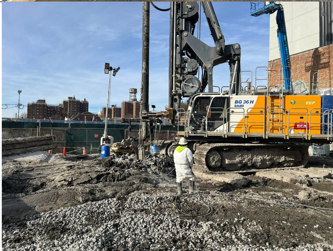
Photo 2- Representative photo of wet mix sample collection.
