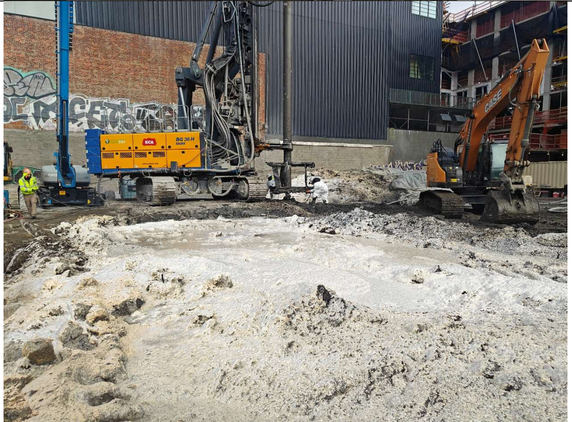
Photo 4- Representative photo of sprayed ISS area after completion of the 2 columns.
