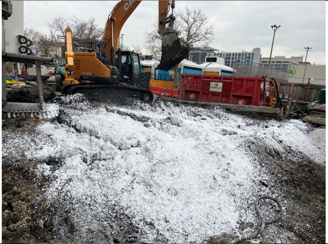
Photo 3- Representative photo ISS installation area during stockpiling.
