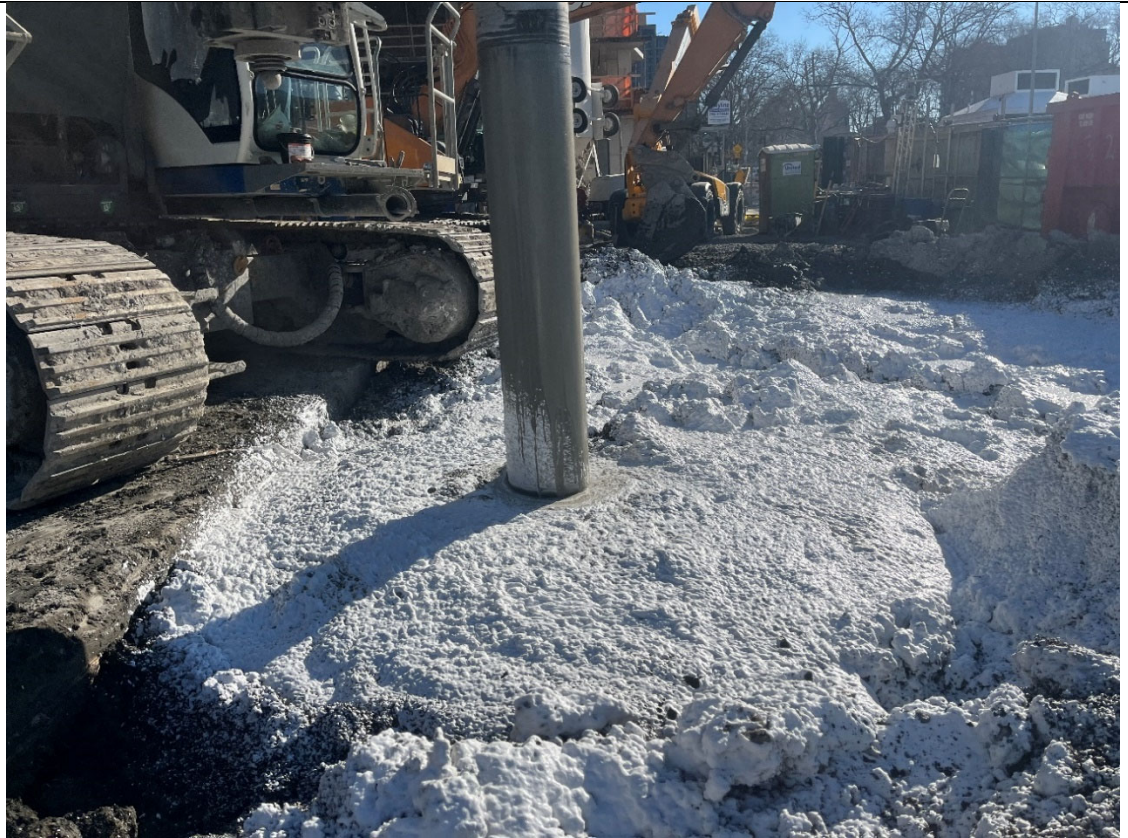
Photo 1- Representative photo of ISS installation.
