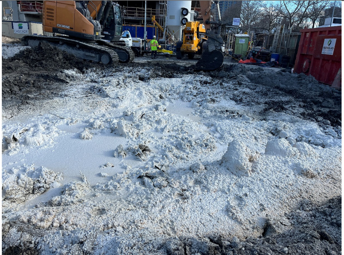
Photo 3- Representative photo of ISS installation area sprayed with Atmos Foam.
