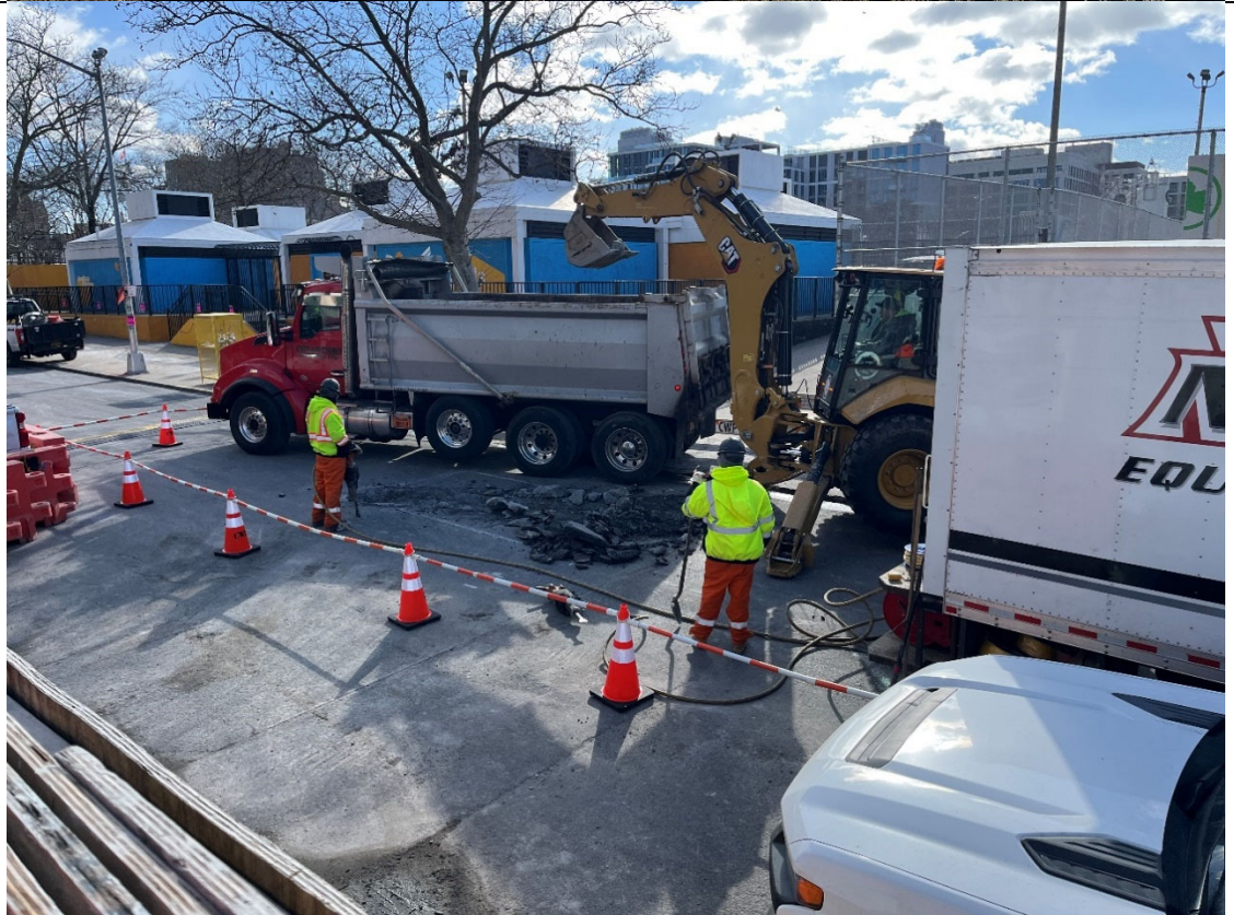
Photo 2- Representative photo of Road work along Douglass Street.
