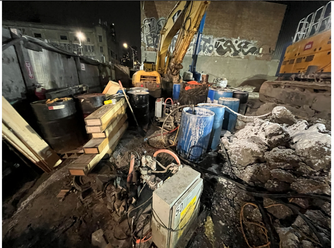
Photo 4- Representative photo of two functional ATMOS foam units on site.
