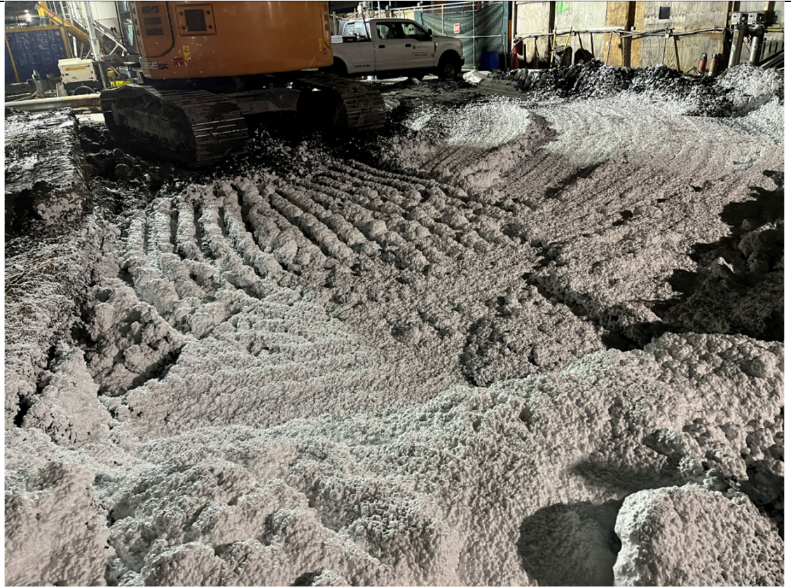
Photo 5- Representative photo of backfilled excavation area covered with ATMOS foam.
