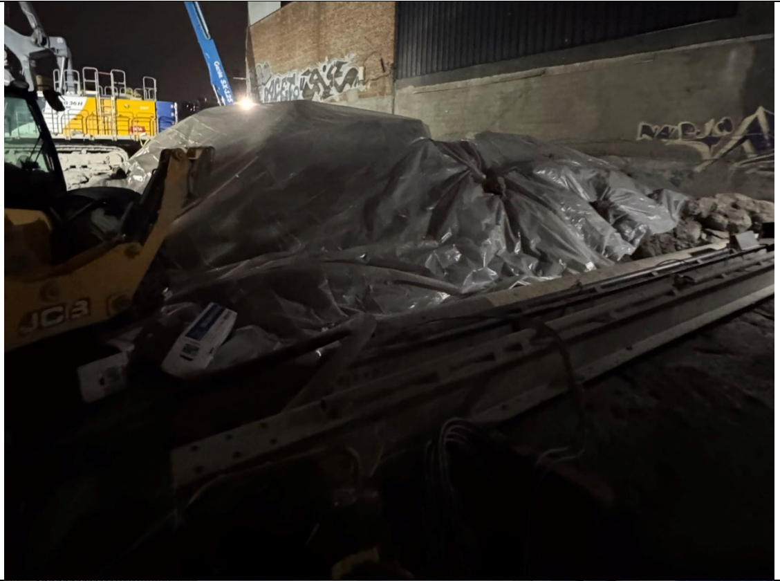
Photo 1- Representative photo of swell stockpiled covered with poly at the end of the day.
