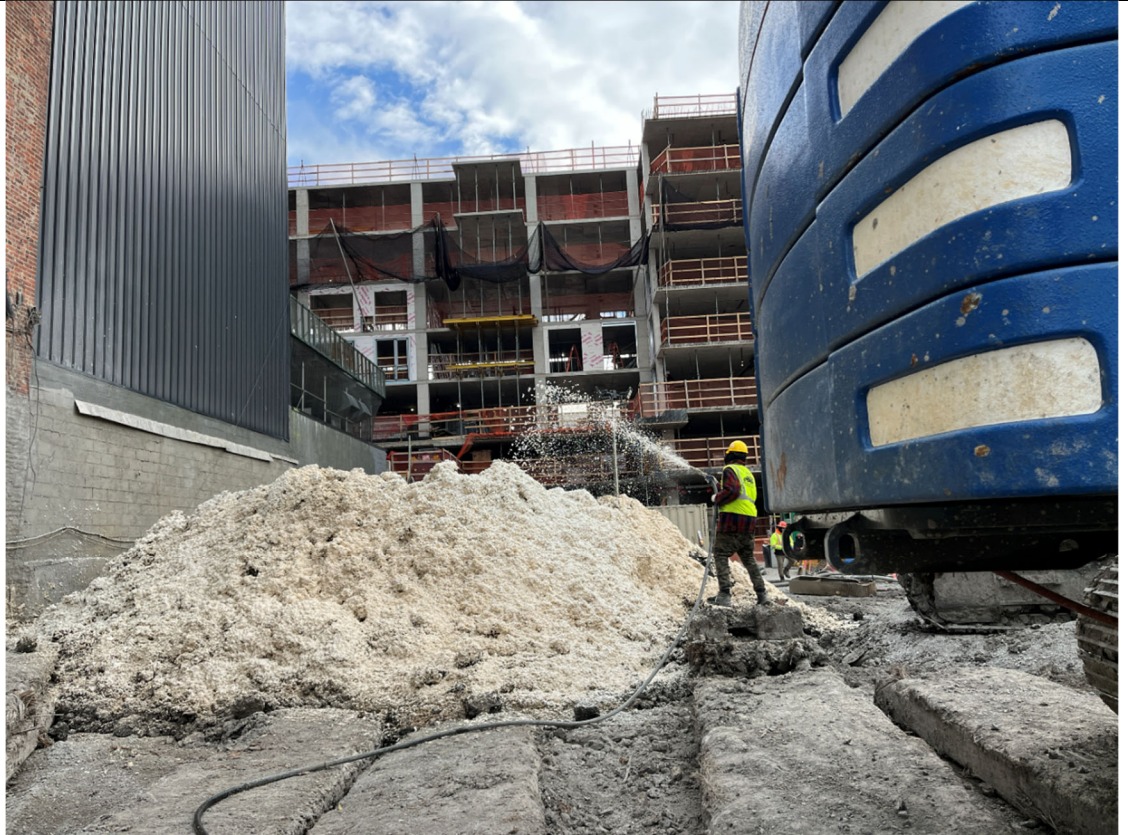
Photo 2- Representative photo of swell stockpile covered with ATMOS foam.
