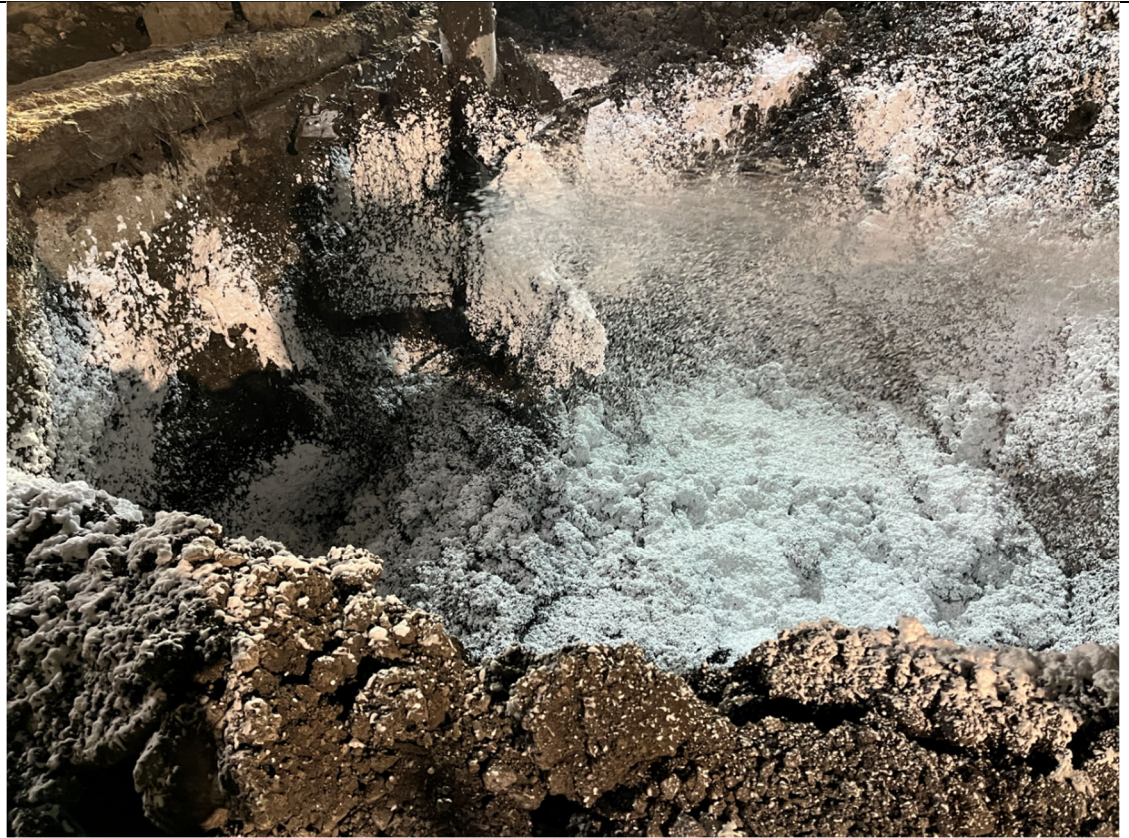
Photo 3- Representative photo of ATMOS foam application during auger retrieval.
