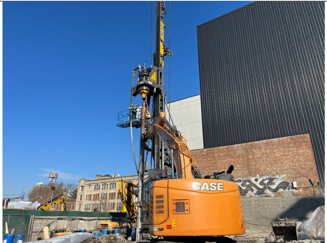
Photo 3- Representative photo of rig maintenance.
