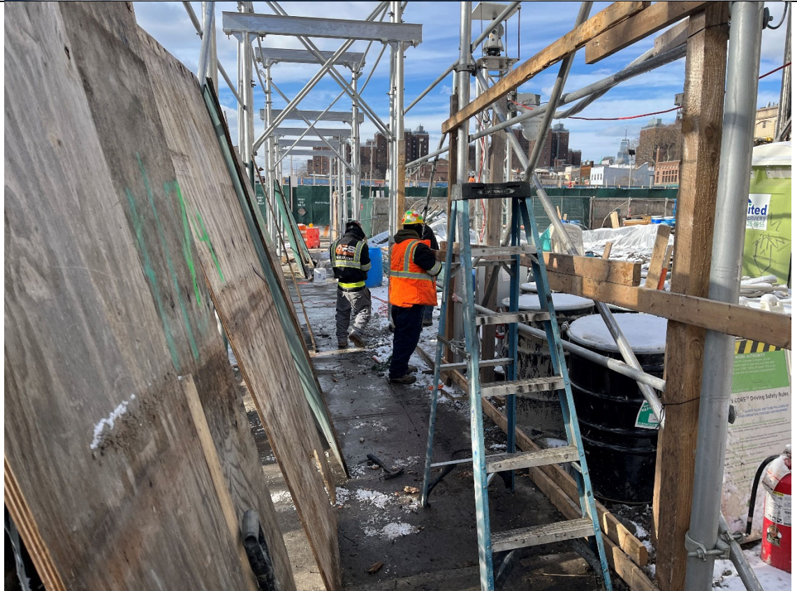
Photo 2- Representative photo of fence and scaffolding work along Douglass St.
