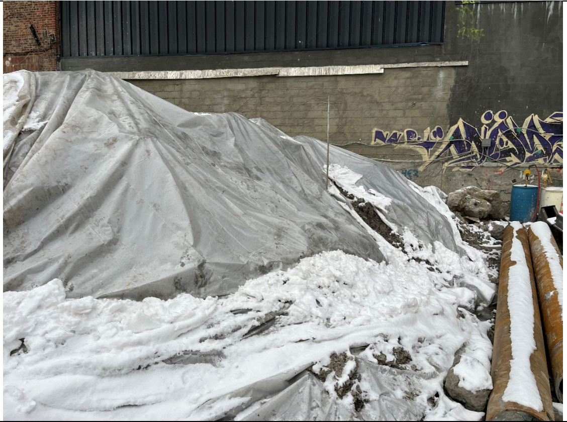
Photo 3- Representative photo of swell stockpile covered in poly.
