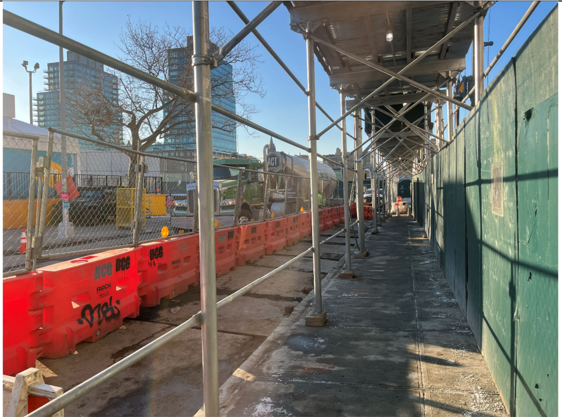
Photo 3- Representative photo of scaffolding.
