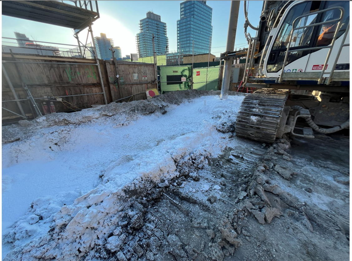
Photo 1- Representative photo of ISS installation.
