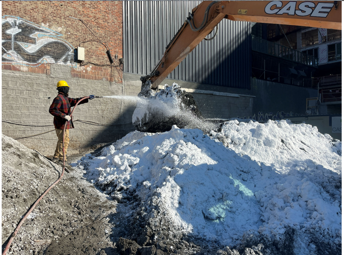
Photo 2- Representative photo of foam application during consolidation of swell material.
