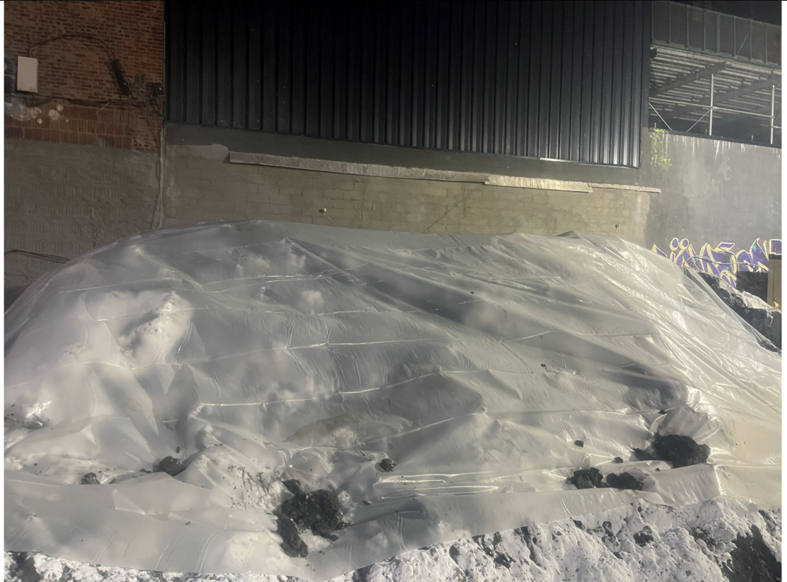
Photo 4- Representative photo of Swell stockpile covered in Atmos Foam at the end of the day.
