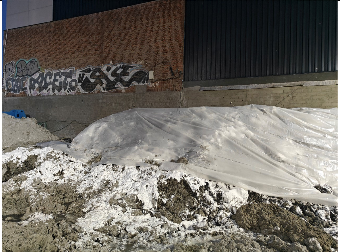
Photo 2- Representative photo of covered swell stockpile.
