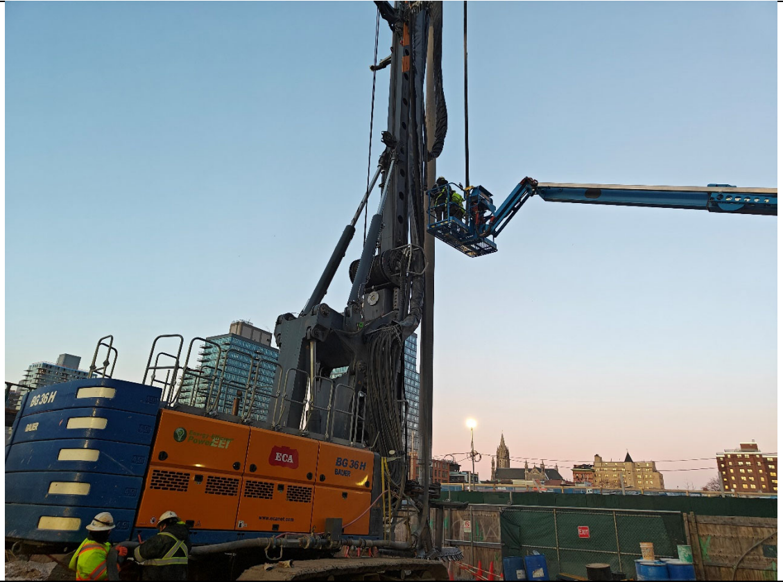
Photo 3- Representative photo of rig maintenance.
