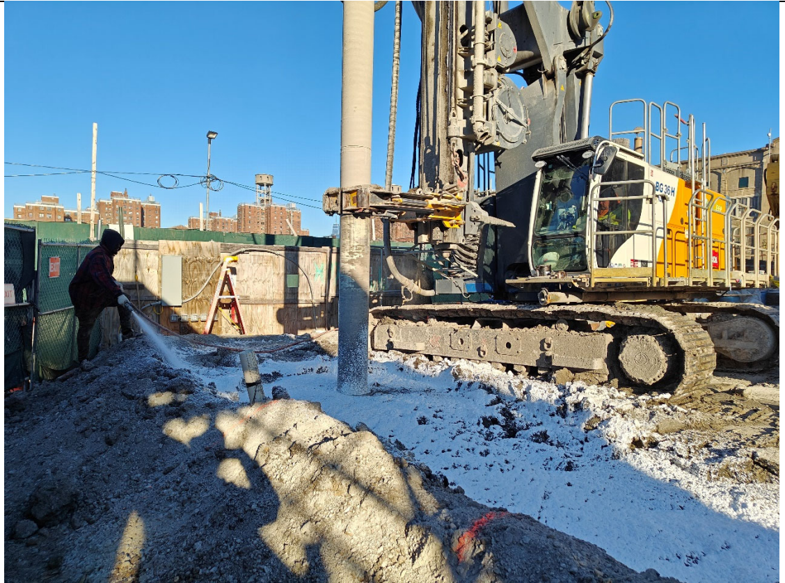
Photo 1- Representative photo of ISS installation and foam application.
