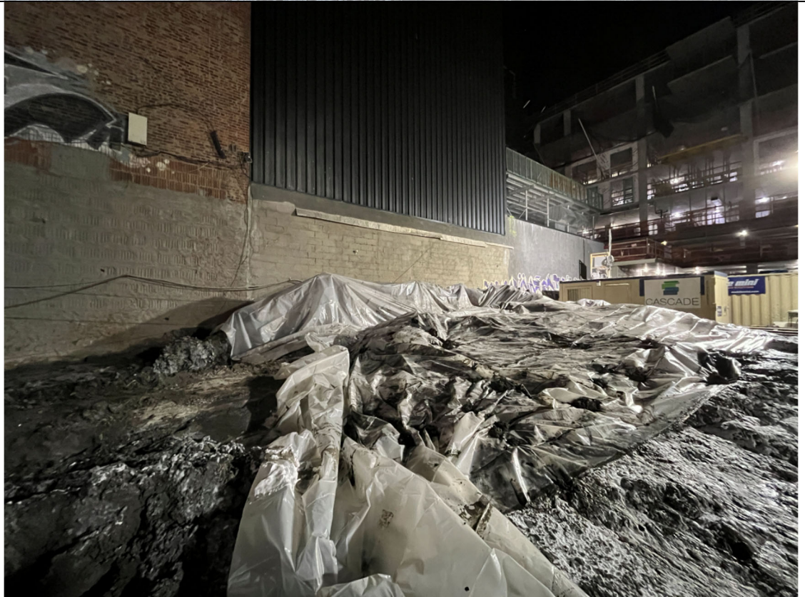
Photo 4- Representative photo of Swell stockpile covered in Atmos Foam and poly at the end of the day.
