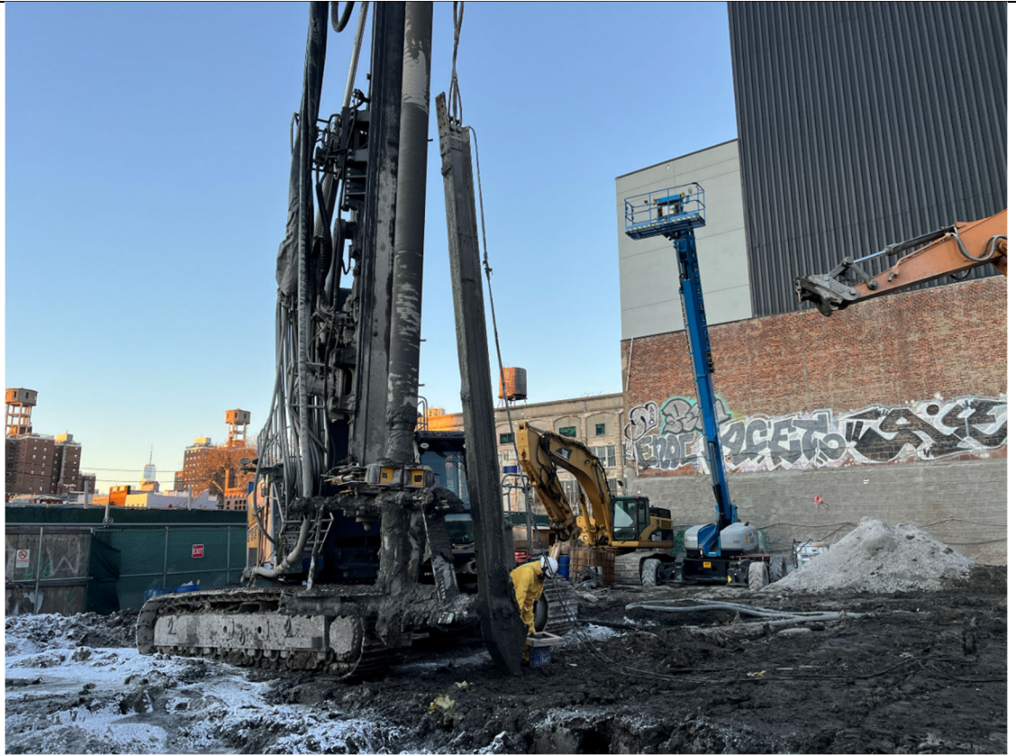
Photo 3- Representative photo of wet mix sample collection.
