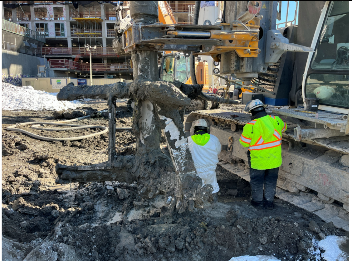
Photo 2- Representative photo of Cascade replacing auger teeth.
