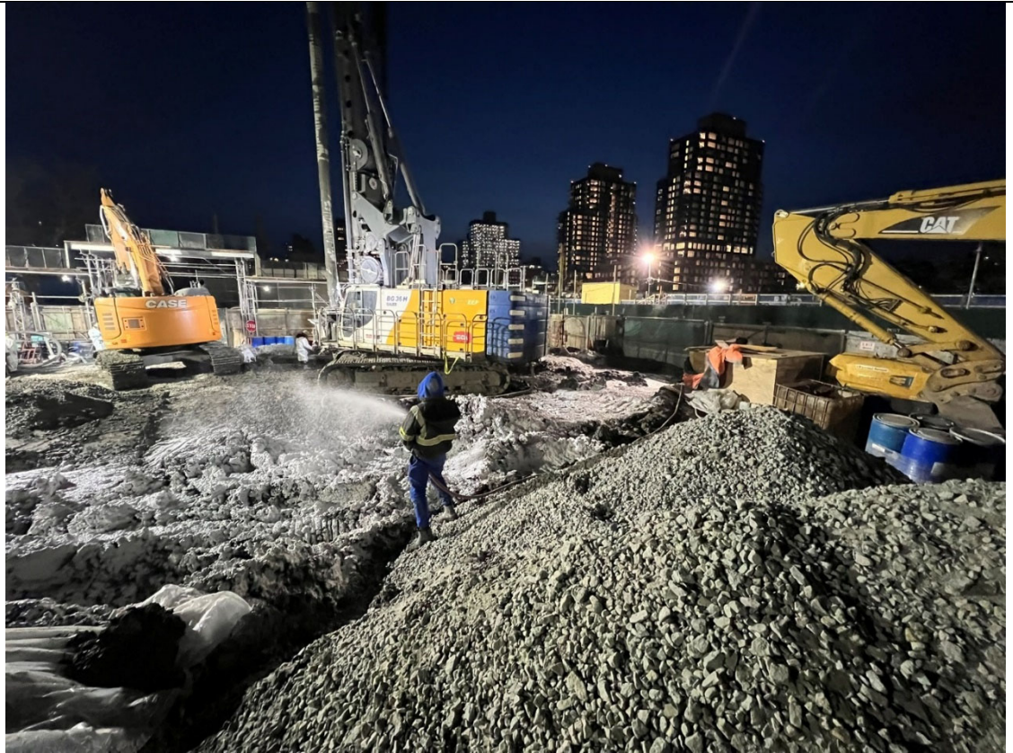
Photo 3- Representative photo of spraying the work area at the end of the day.
