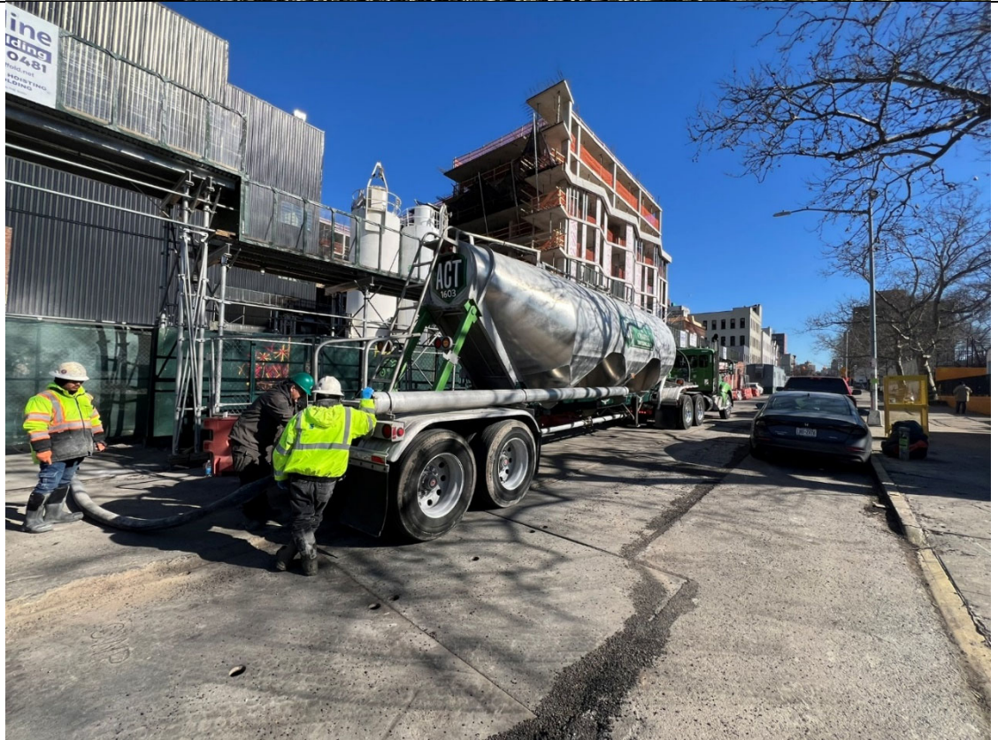
Photo 4- Representative photo of a slag delivery.
