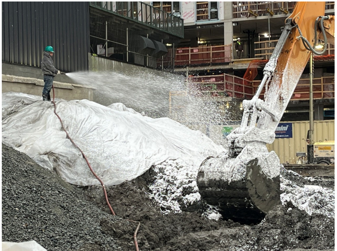
Photo 2- Representative photo of spraying Atmos Foam on stockpile while trucking.
