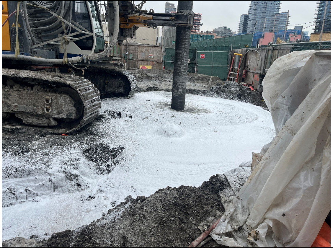
Photo 1- Representative photo of ISS installation.
