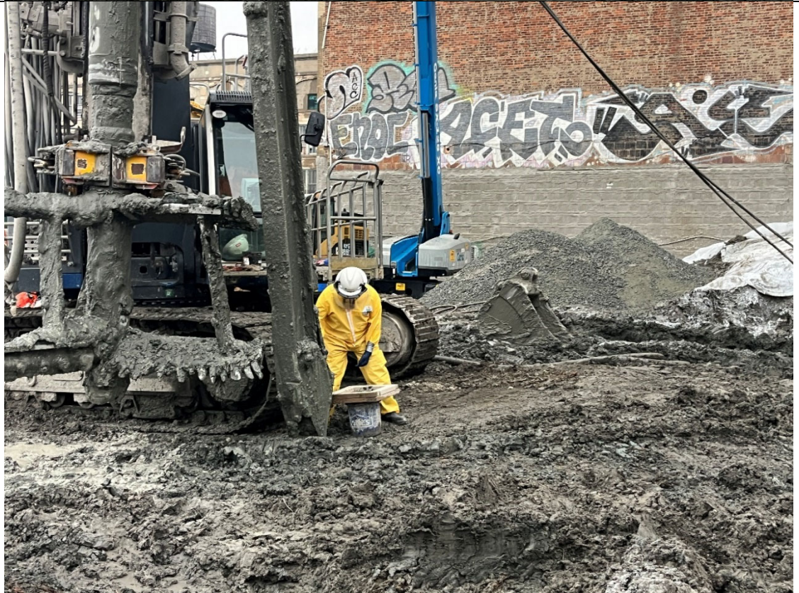
Photo 4- Representative photo of wet mix sample collected from column 130.
