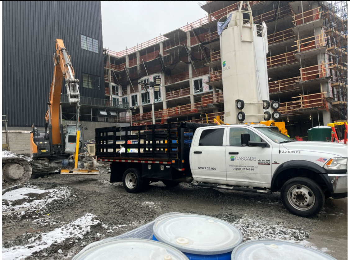
Photo 2- Representative photo of Cascade demobilizing equipment.
