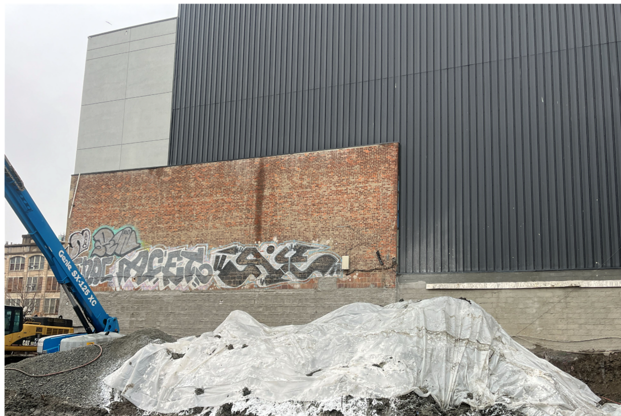
Photo 4- Representative photo of swell stockpile covered with poly.
