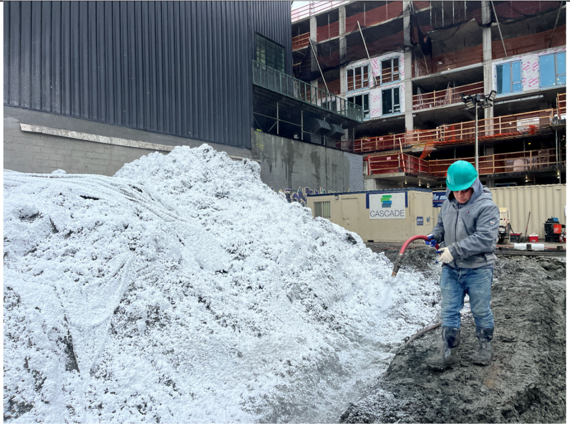
Photo 3- Representative photo of swell stockpile covered with ATMOS foam.
