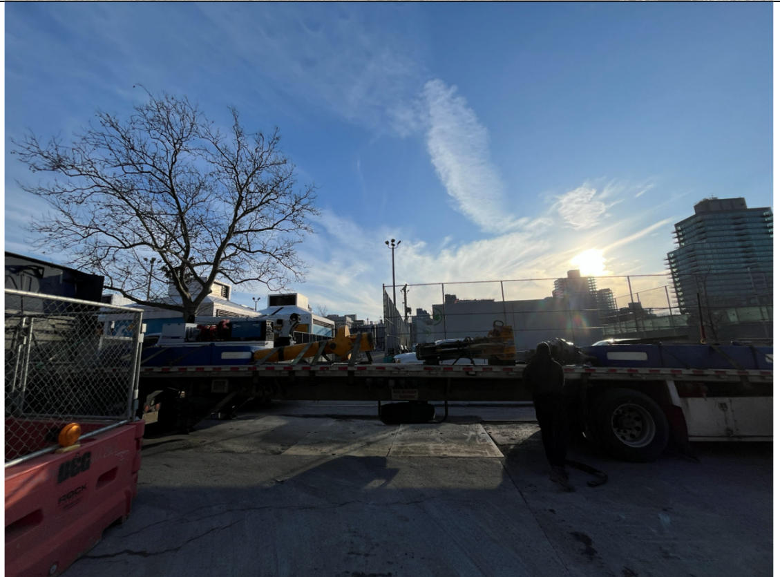
Photo 2- Representative photo of Cascade demobilizing equipment.
