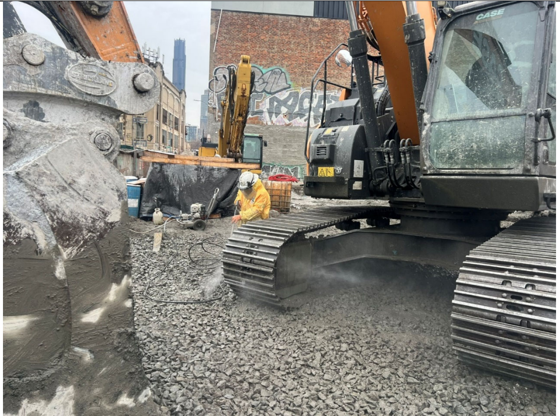
Photo 3- Representative photo of the excavator being washed.
