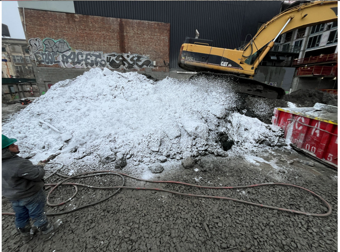
Photo 4- Representative photo of foam application to swell material.
