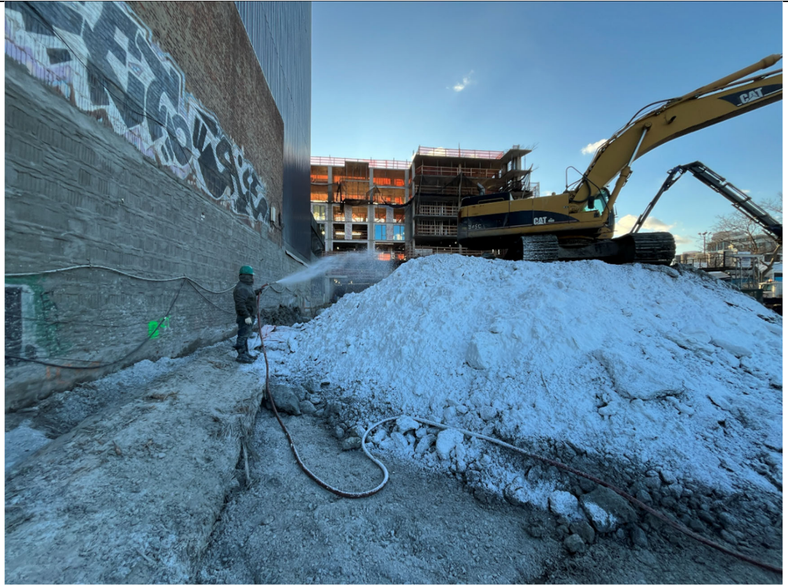
Photo 3- Representative photo ATMOS foam application.
