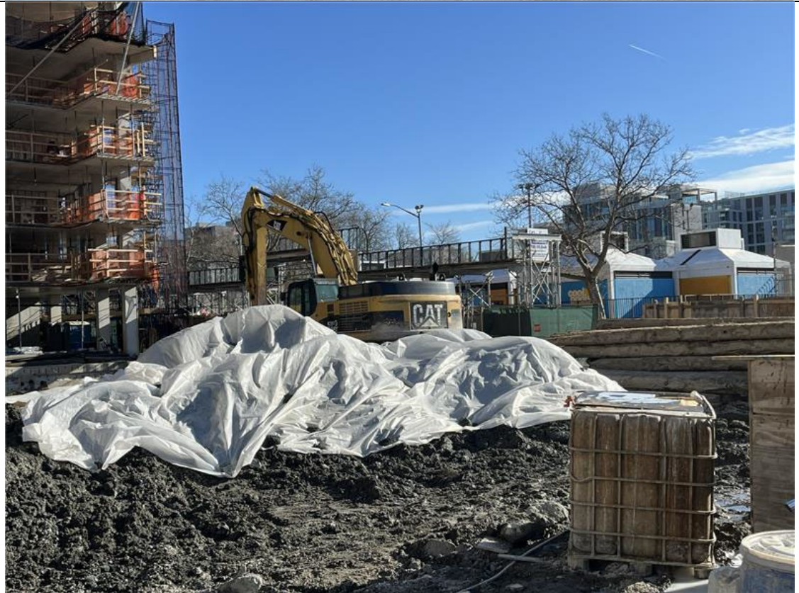
Photo 4- Representative photo of the treated material stockpile covered with poly.
