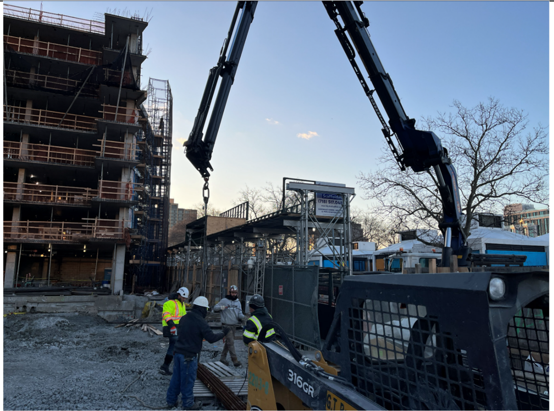
Photo 1- Representative photo of rebar delivery.
