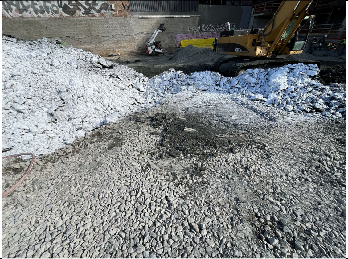
Photo 3- Representative photo of sprayed stockpile.
