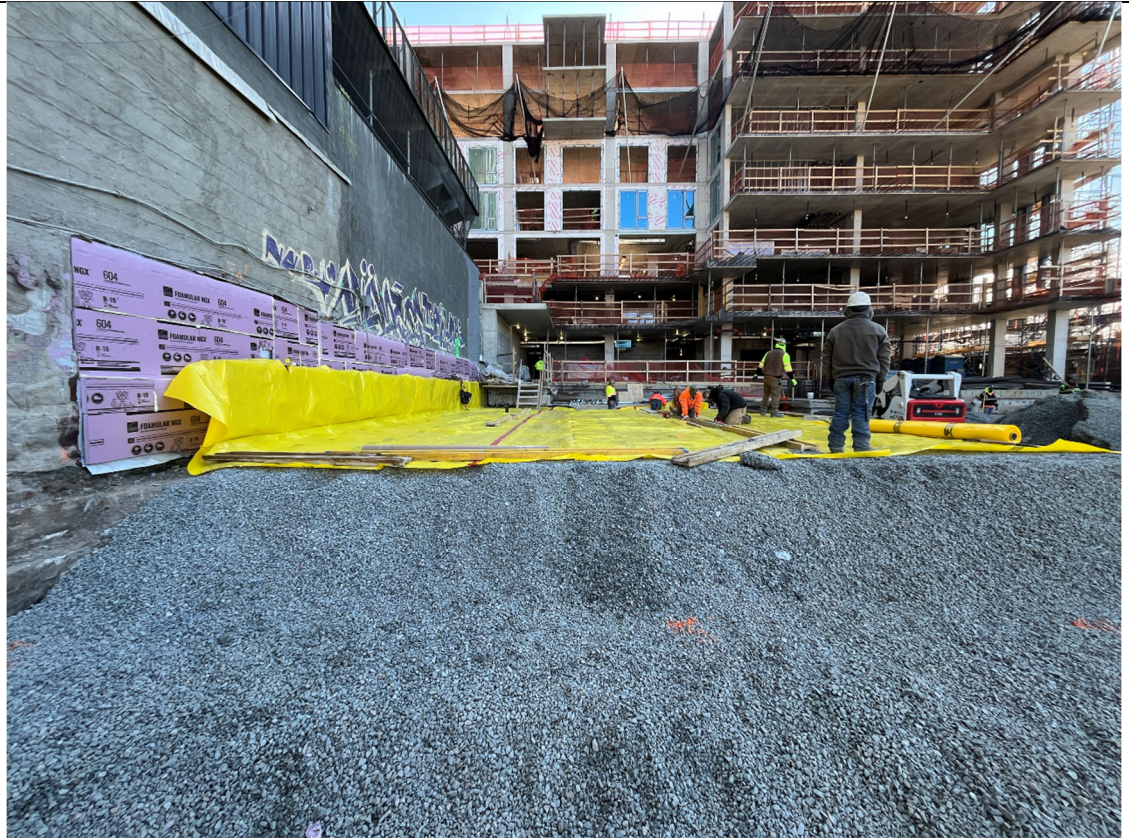
Photo 1- Representative photo of vapor barrier installation in progress.
