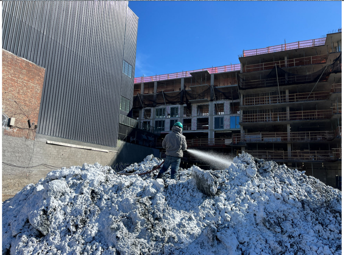
Photo 2- Representative photo of spraying treated material stockpile.
