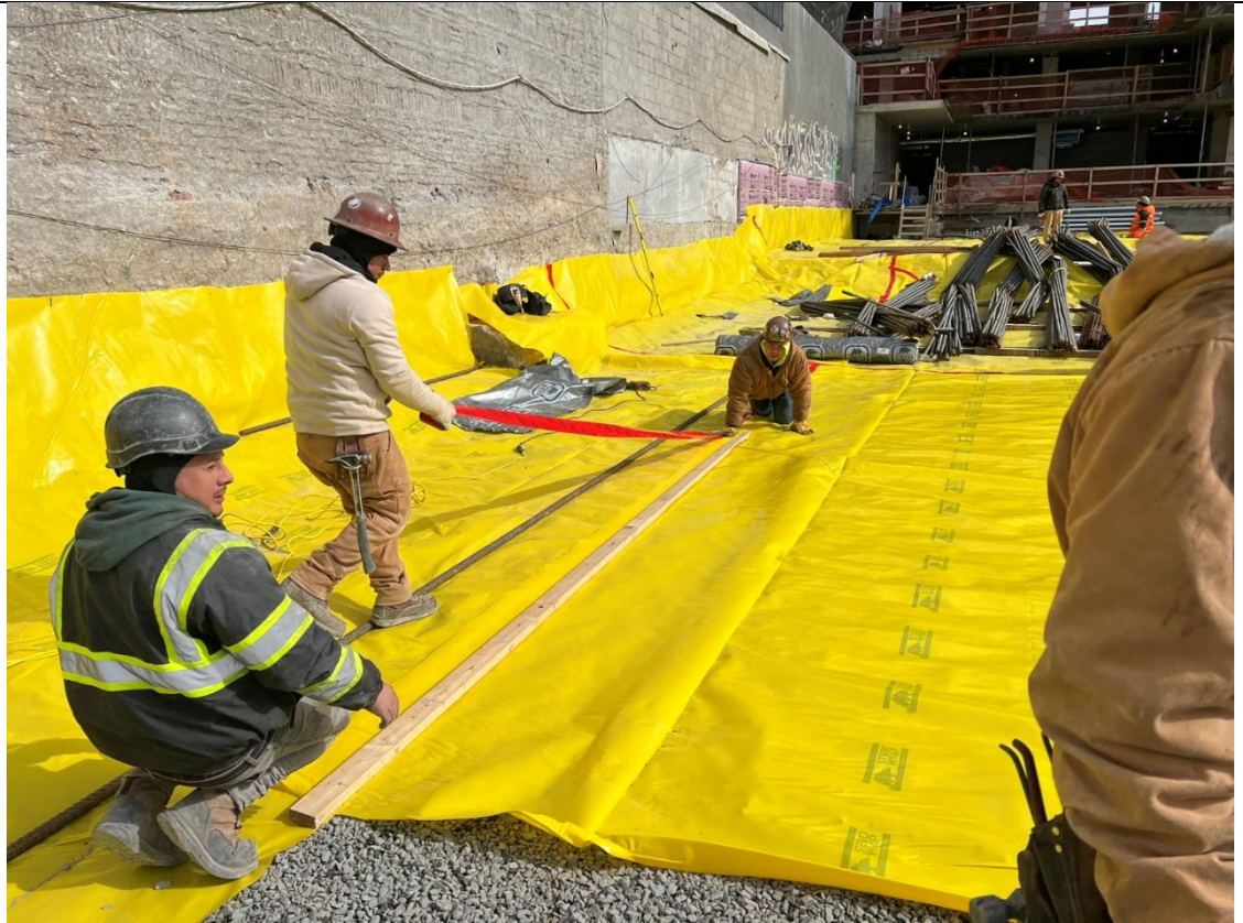
Photo 3- Representative photo of vapor barrier installation.
