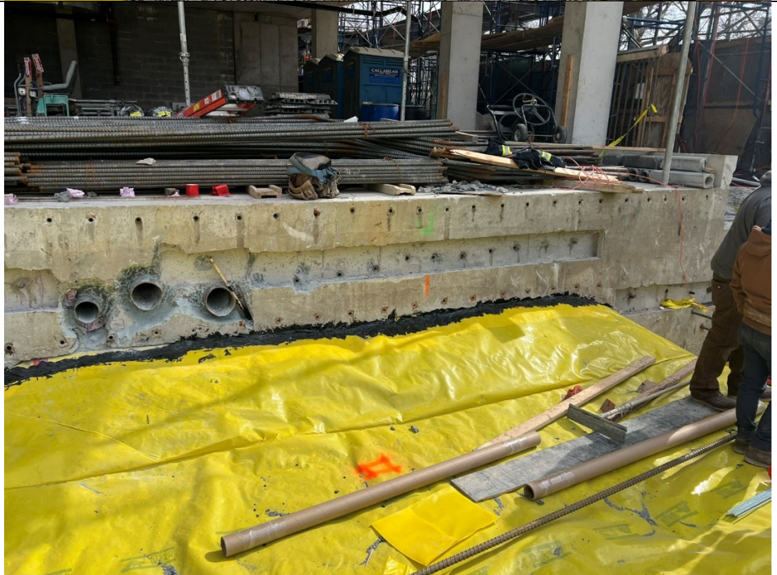
Photo 4- Representative photo of the vapor barrier.
